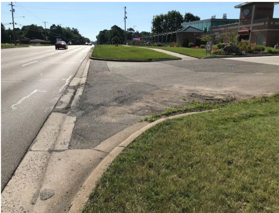
Drive & Shine's west drive (east-facing): the contoured curb and the lack of a visible sign encourages eastbound vehicles to enter.
