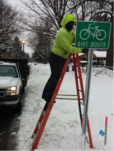
Bicycle route signage
