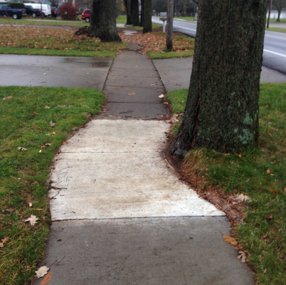
~300 spot repairs of concrete, sidewalk slabs
