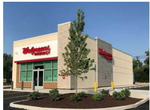
Note: high quality building materials, modern design, sidewalks to parking areas, and landscaping
