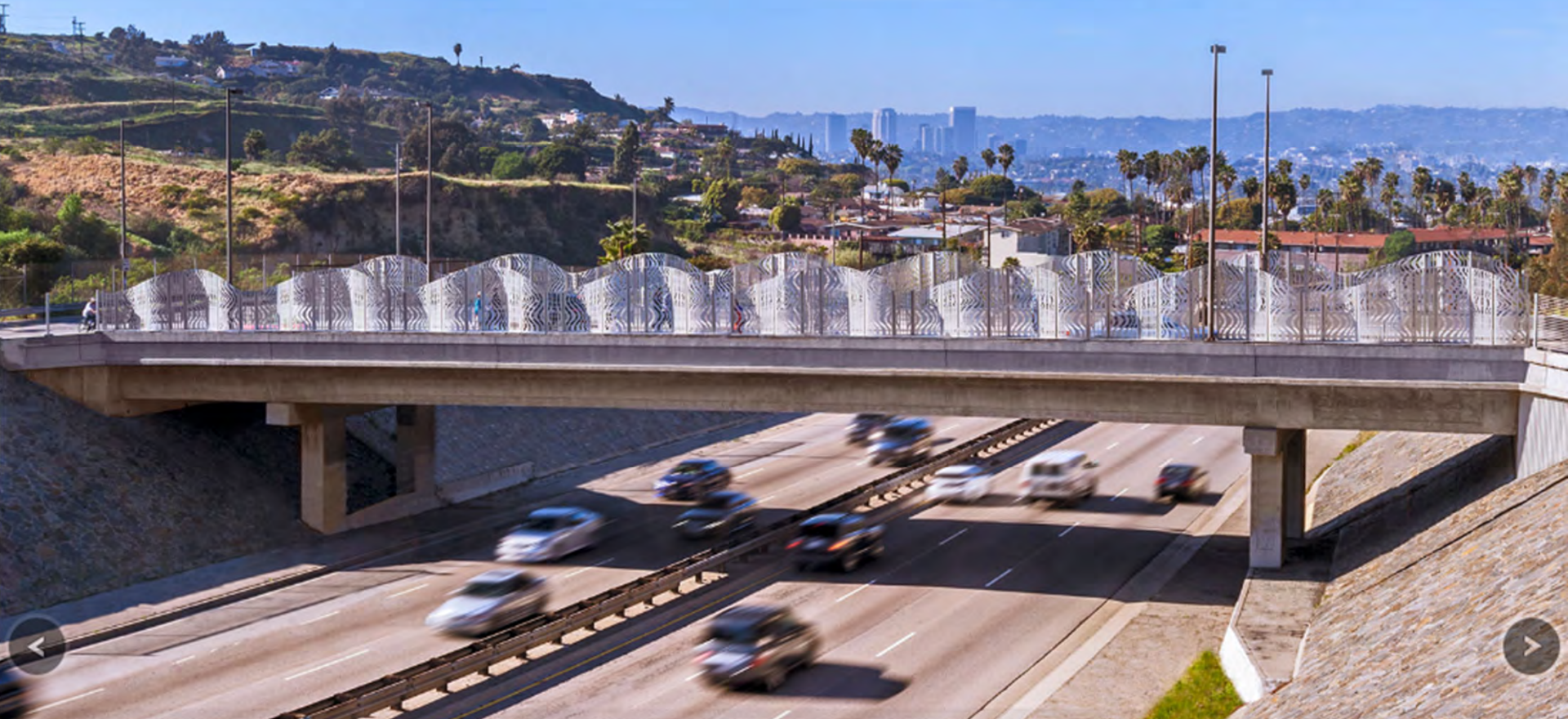
2012 / BALDWIN HILLS GATEWAY / Ken Hahn Bridge, Los Angeles, California
