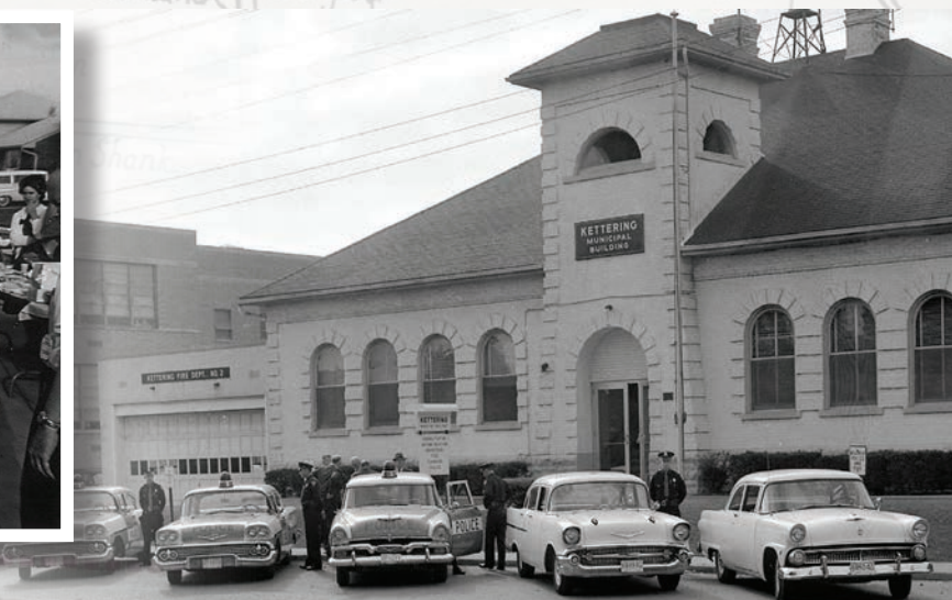
1960 Police Car inspection at Original Municipal Building
