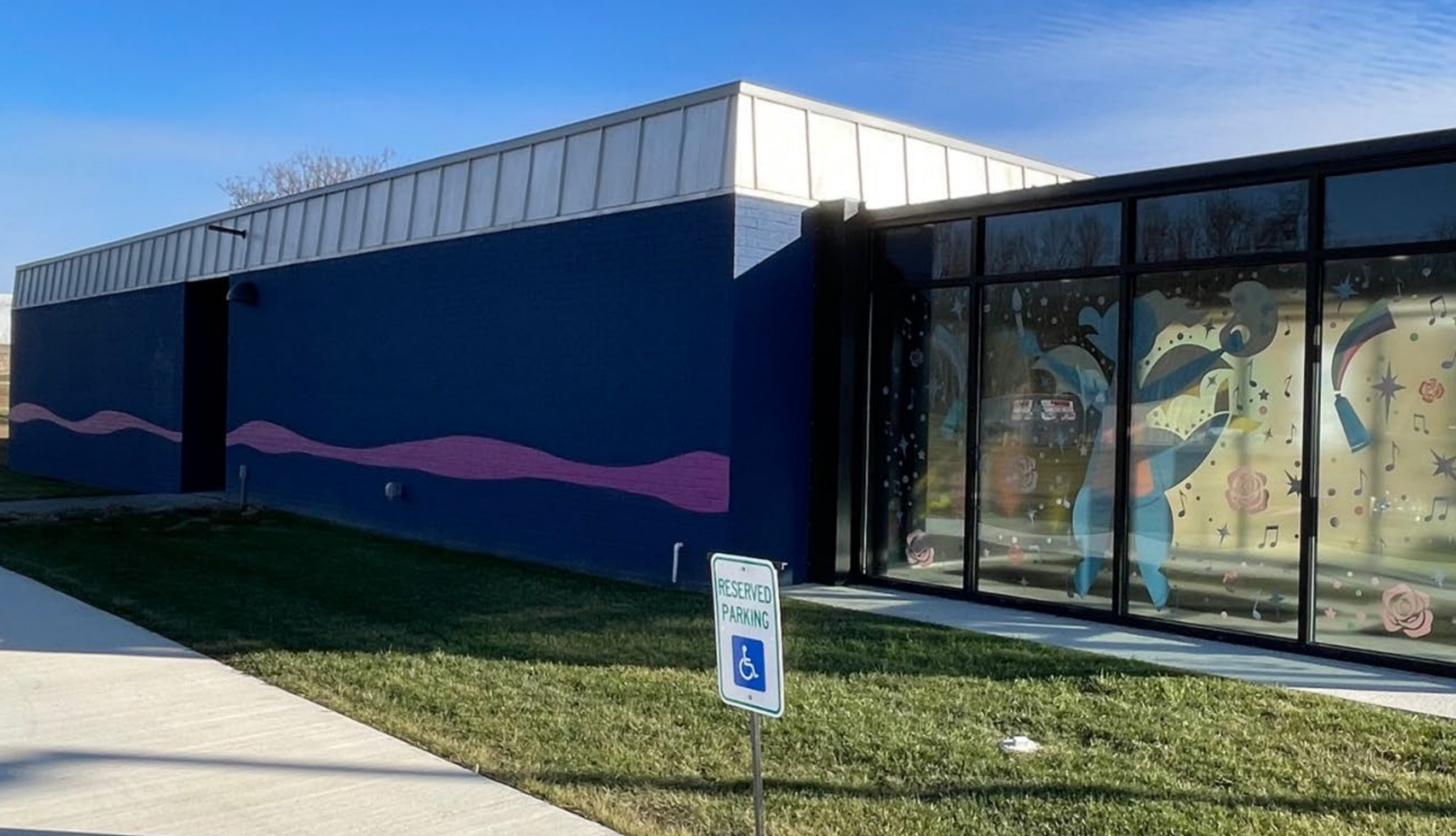
VIEW OF FRONT ENTRANCE + SIDE WALL
