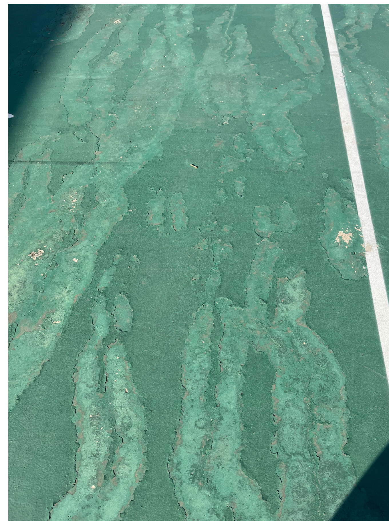
EXISTING SHUFFLEBOARD SURFACE
