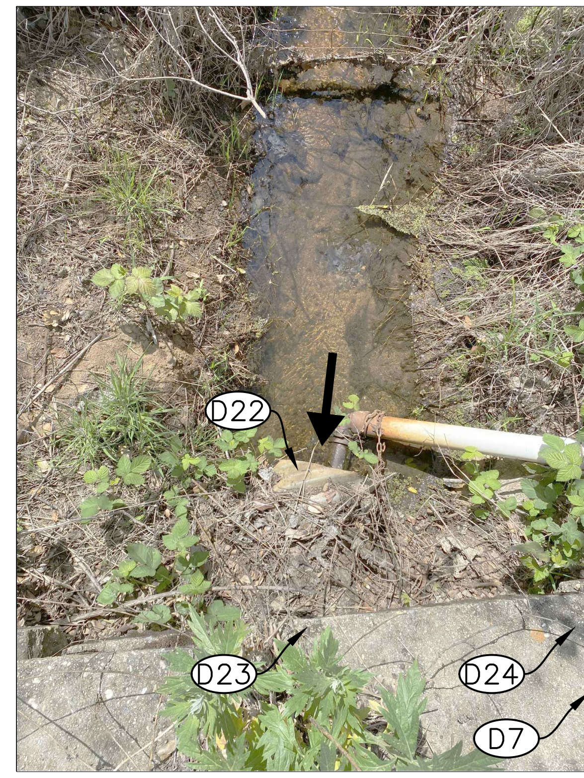
CULVERT INLET LOCATED EAST OF LAIRD ROAD (LOOKING EAST)
