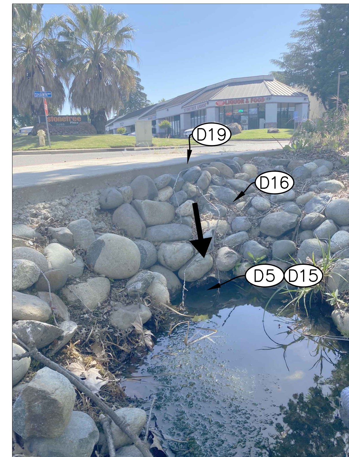
OUTFALL LOCATED SOUTH OF SHAWN WAY RD (LOOKING NORTH)
