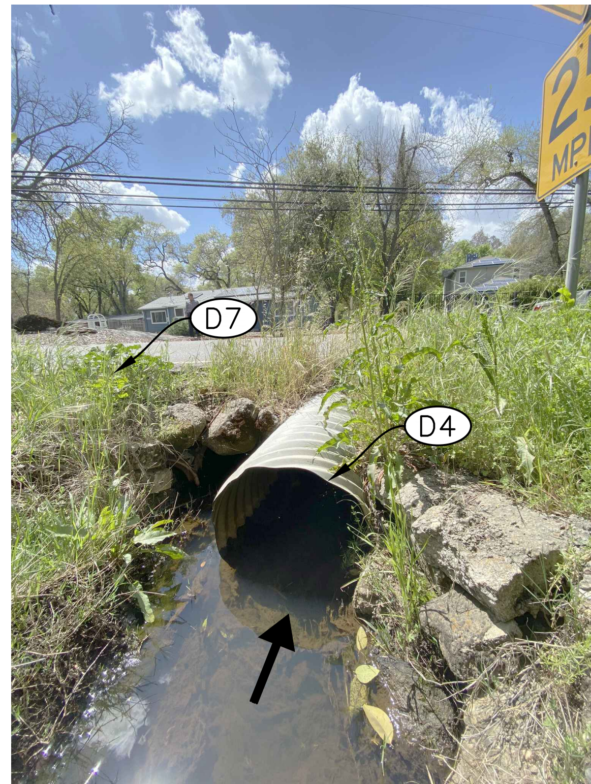
CULVERT INLET LOCATED EAST OF HORSESHOE BAR ROAD (LOOKING WEST)
