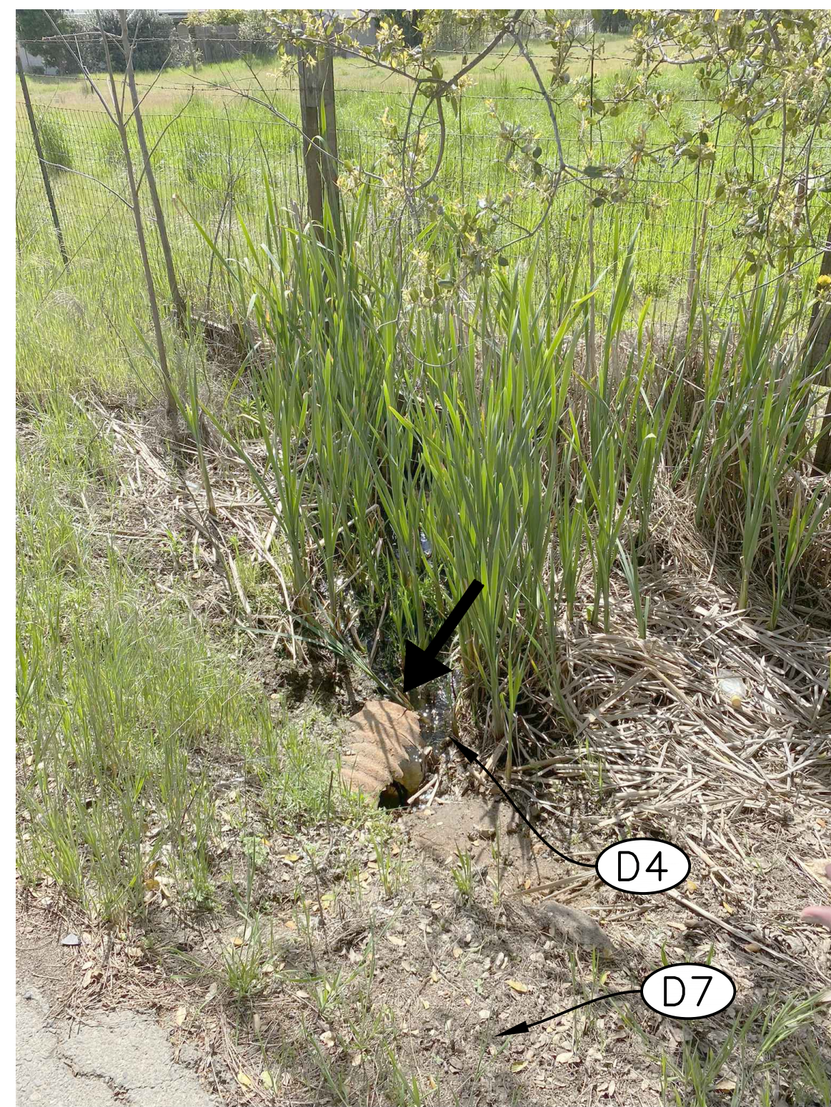
CULVERT INLET LOCATED WEST OF DELMAR AVENUE (LOOKING WEST)
