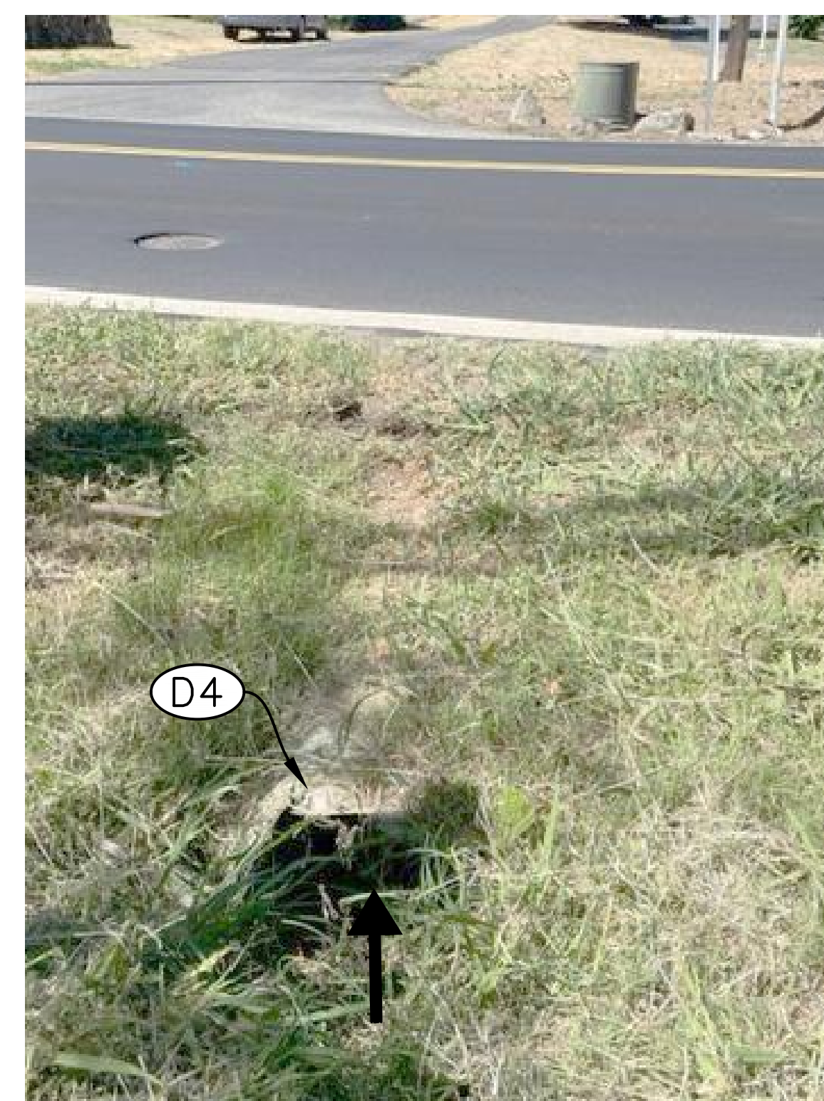
CULVERT INLET LOCATED EAST OF LAIRD ROAD (LOOKING WEST)
