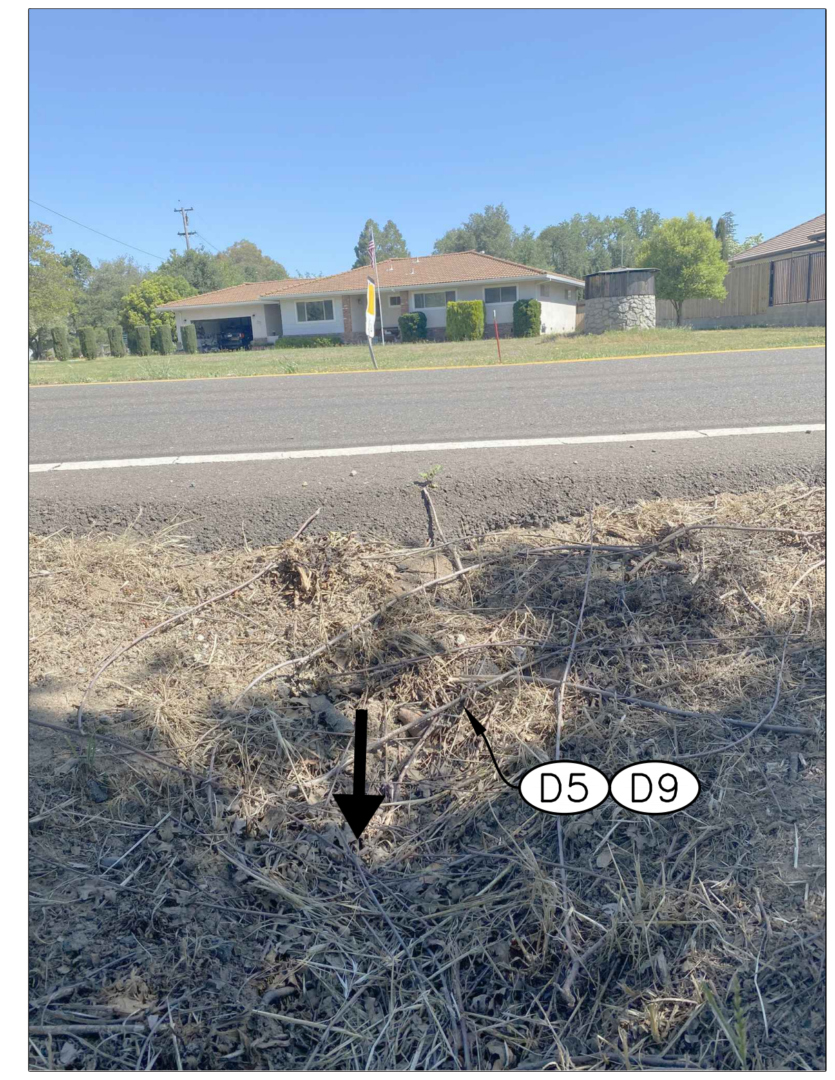
CULVERT OUTFALL LOCATED SOUTH OF BRACE ROAD (LOOKING NORTH)
