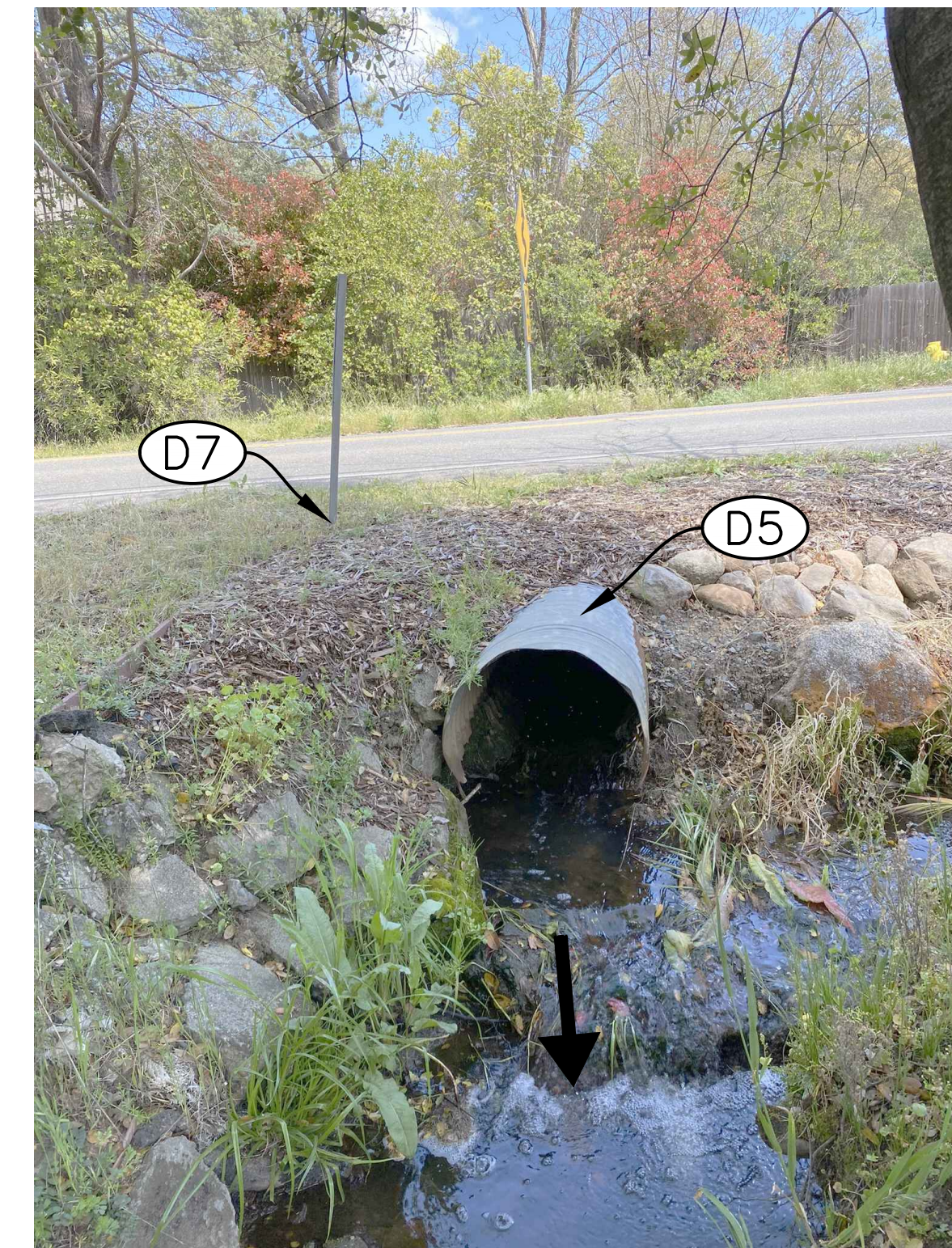
CULVERT OUTFALL LOCATED WEST OF HORSESHOE BAR ROAD (LOOKING EAST)
