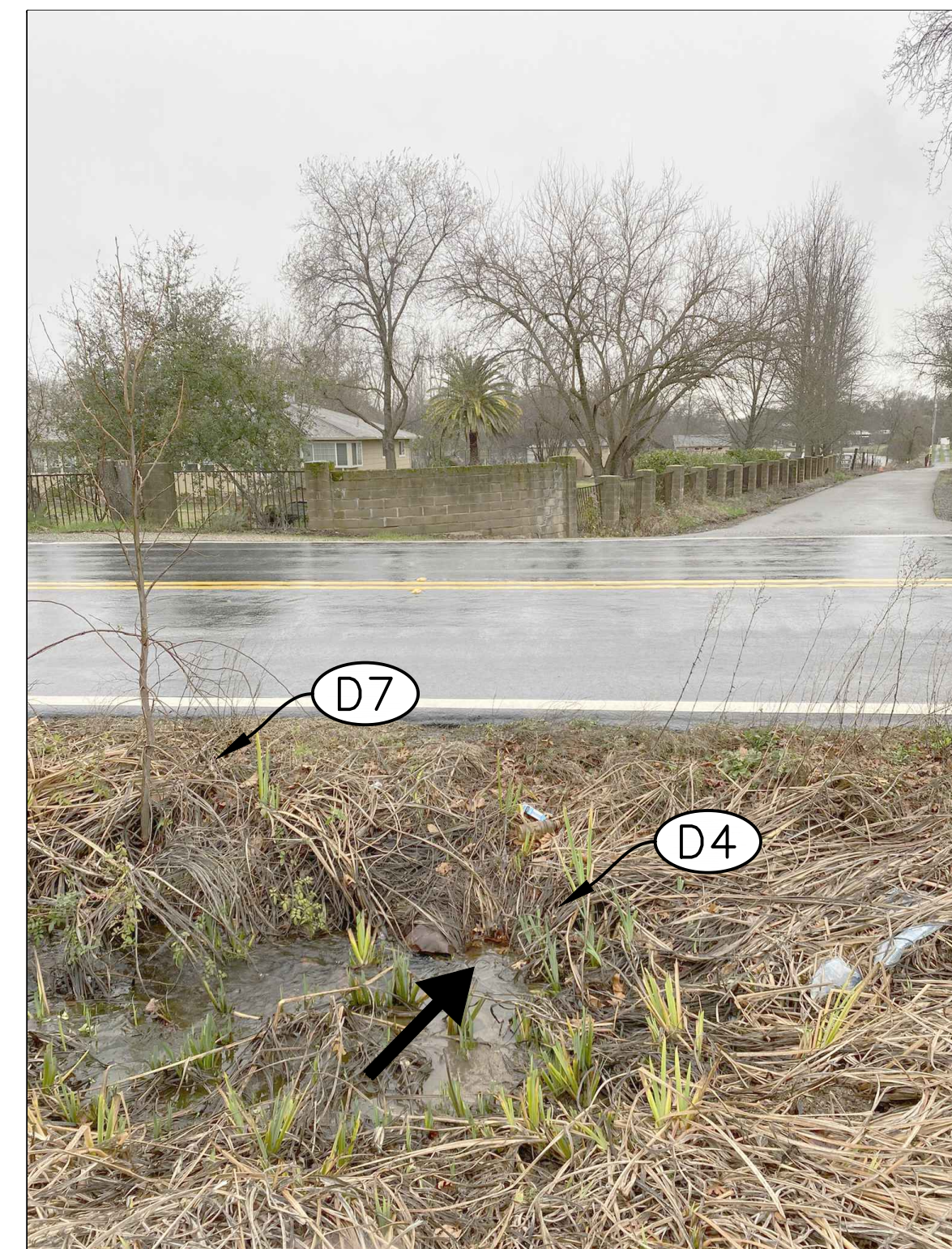
CULVERT INLET LOCATED EAST OF LAIRD ROAD (LOOKING WEST)
