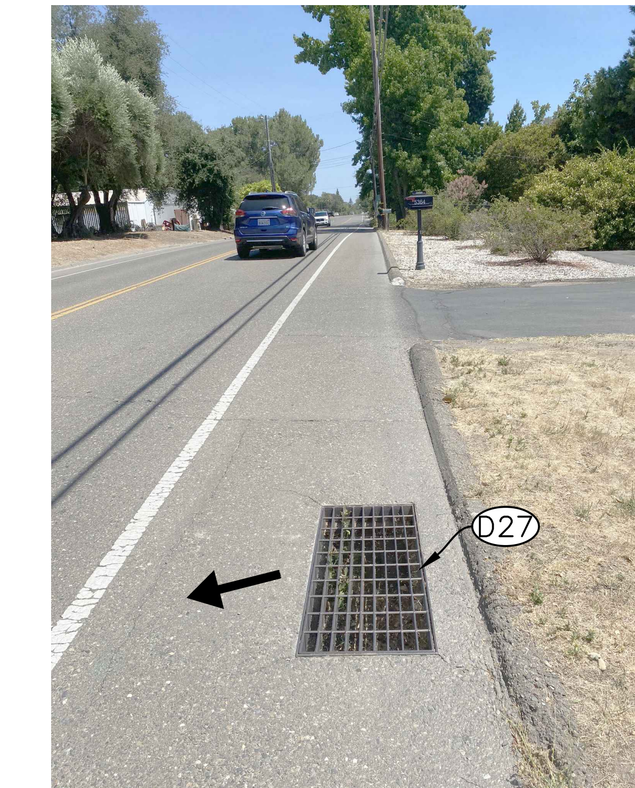
CATCH BASIN SOUTH OF KING (LOOKING EAST)
