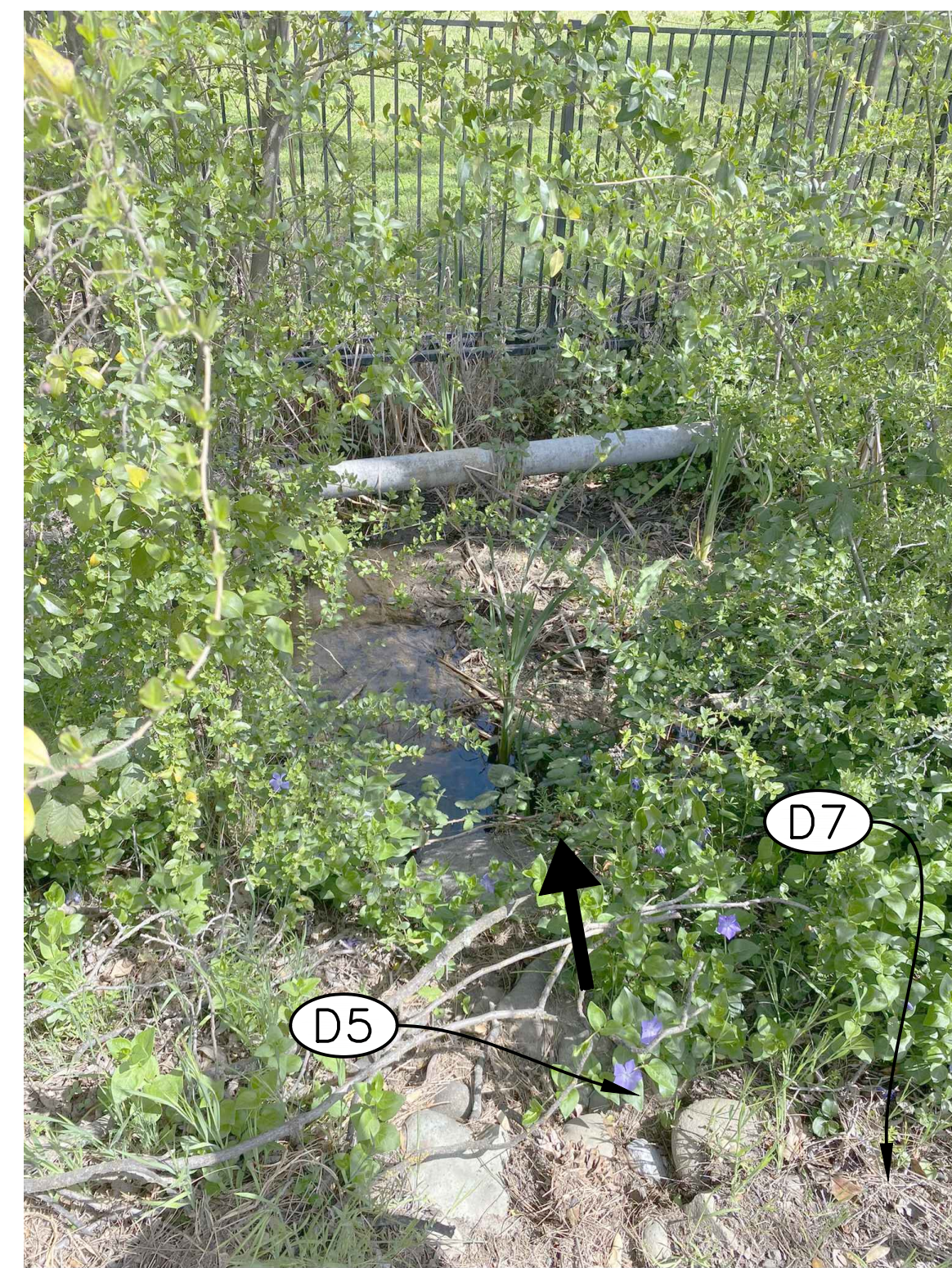
CULVERT OUTFALL LOCATED EAST OF DELMAR AVENUE (LOOKING EAST)
