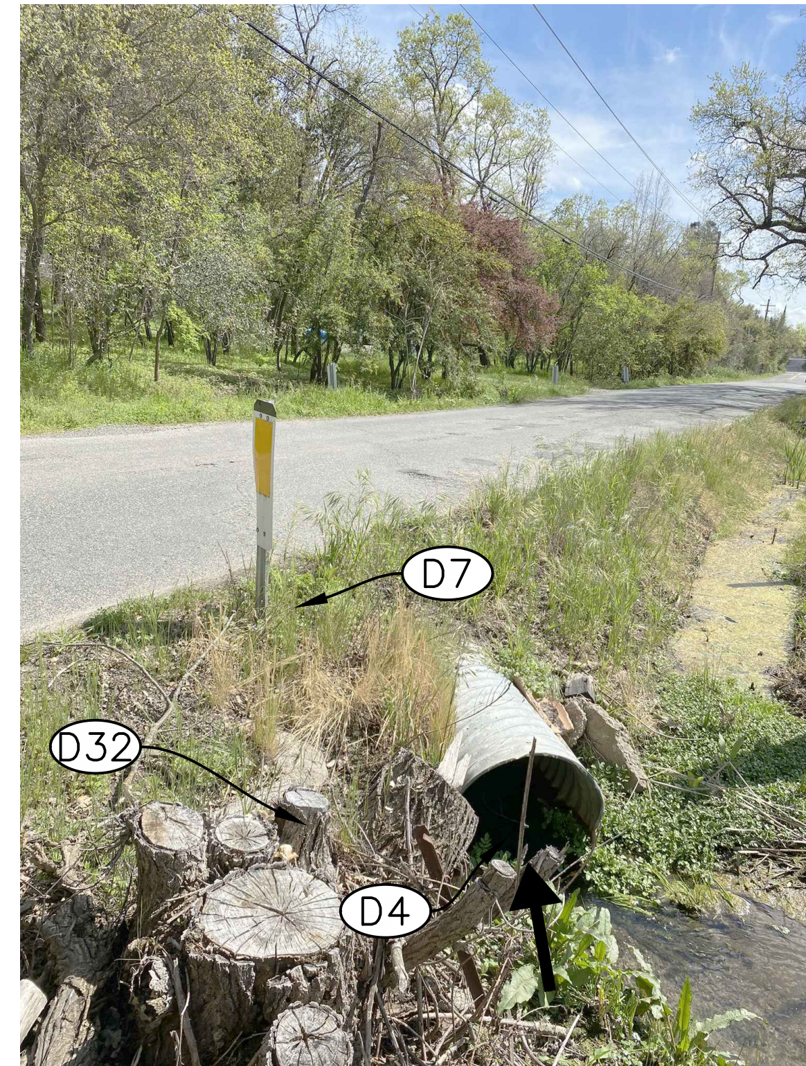
CULVERT INLET LOCATED WEST OF DELMAR AVENUE (LOOKING EAST)
