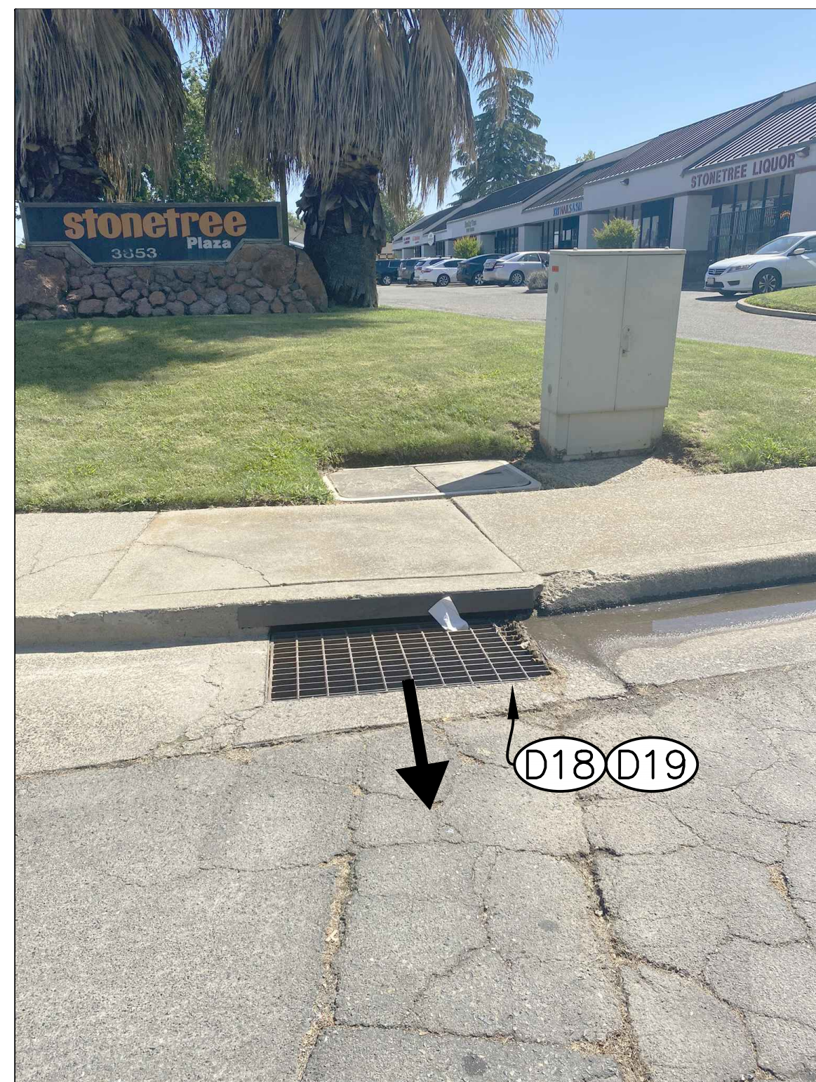
STRUCTURE LOCATED NORTH OF SHAWN WAY RD (LOOKING NORTH)
