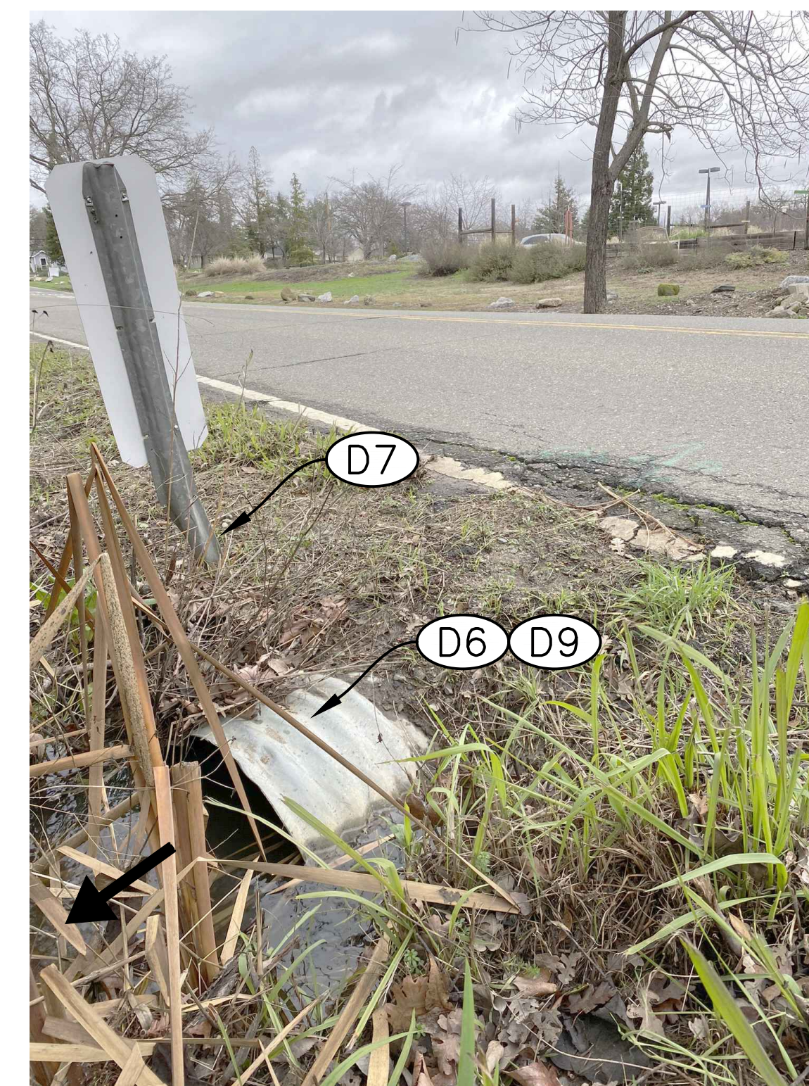
WEST OUTFALL LOCATED EAST OF BARTON ROAD (LOOKING EAST)
