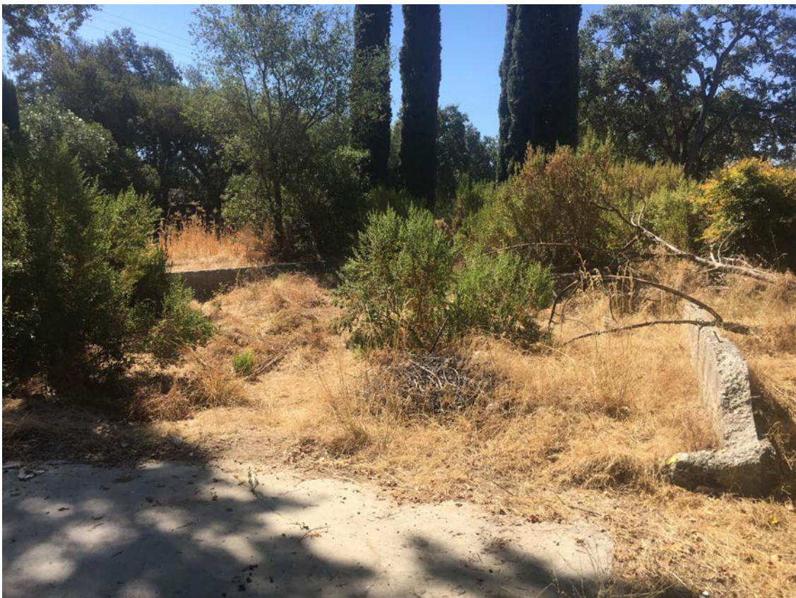
Figure 7. 4105 Starlight Lane House Foundations, looking south.
