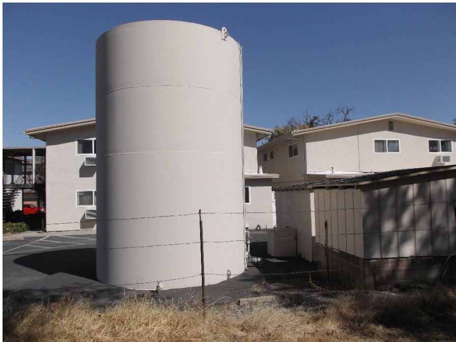
Off-Site water AST located adjacent to northern Site boundary.
