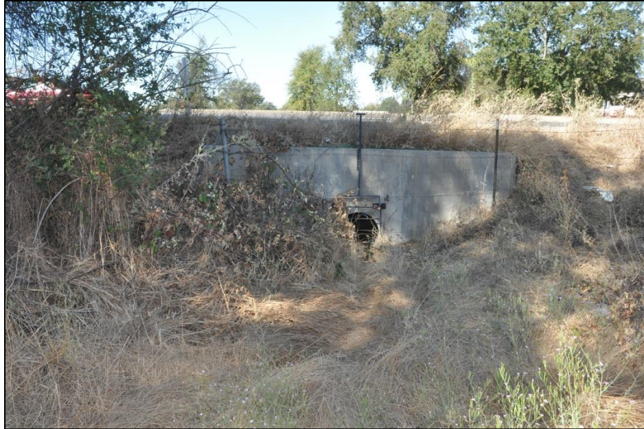
Photograph 7: Culvert from swale in center of Project site allowing flow of water off the Project site to the west under Sierra College Blvd.
