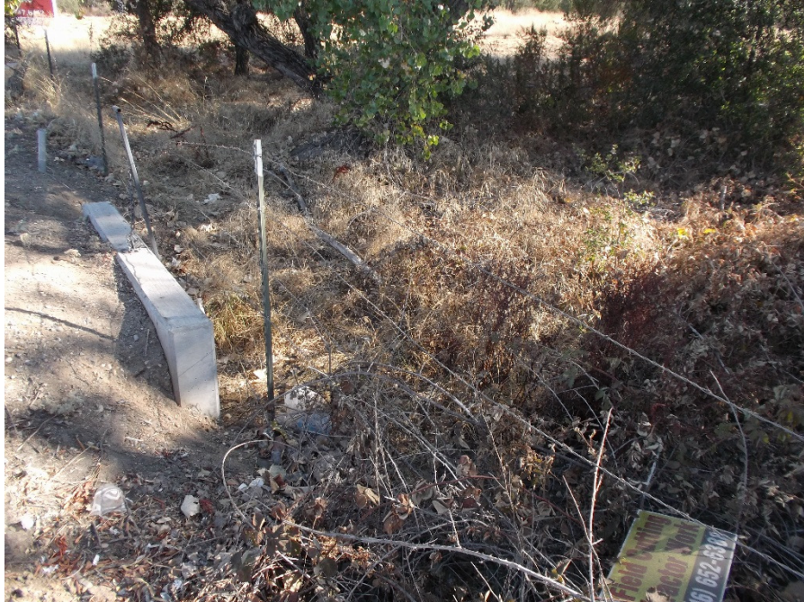
Culvert near southwestern corner of the Site.
