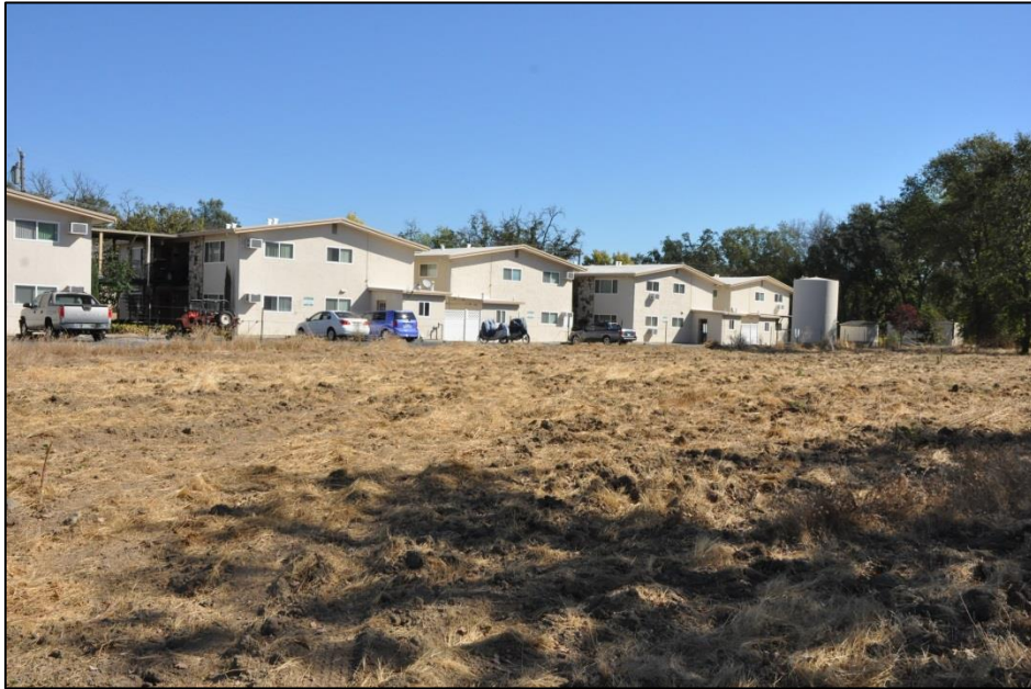
Photograph 1: Small apartment complex to the north of the Project site. View facing north.
