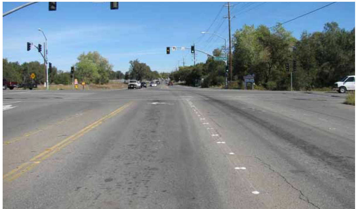
West Gateway Existing Conditions
