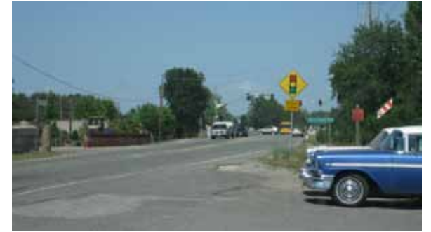
Taylor West Existing Condition
