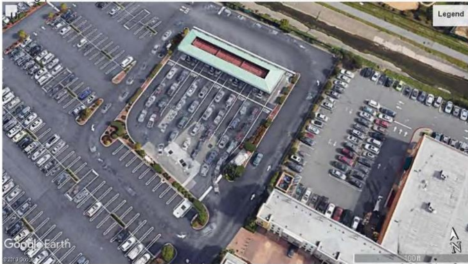
Photo 2: South San Francisco Costco Fueling Facility.
