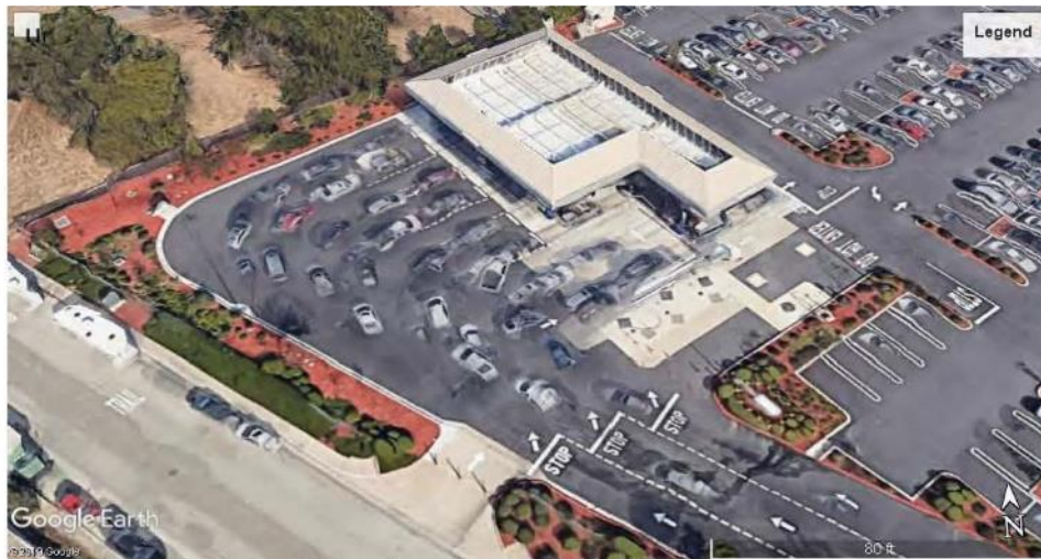
Photo 7: Albany CA Costco Fueling Facility
