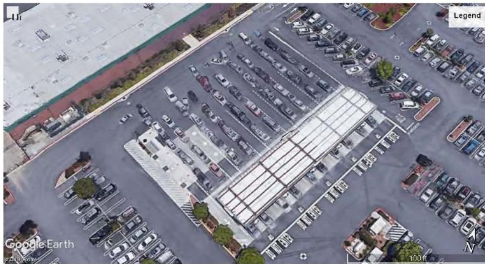
Photo 5: Redwood City Costco Fueling Facility
