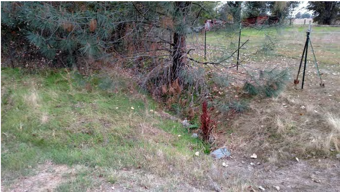
Roadside Ditch (RD-1), facing southwest – 21 November 2018
