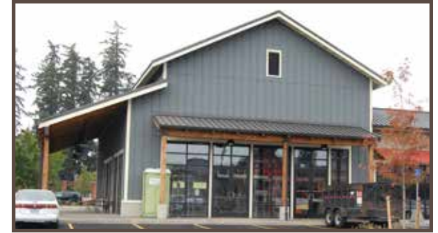
Figure 4.7 - Commercial Gable Roof.
