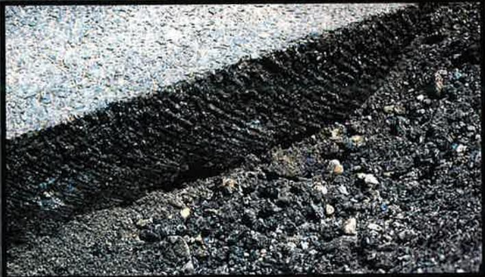
*University research has shown that the Zipper edge improves patch joint bond strength by 25 percent over a saw-cut edge.*
