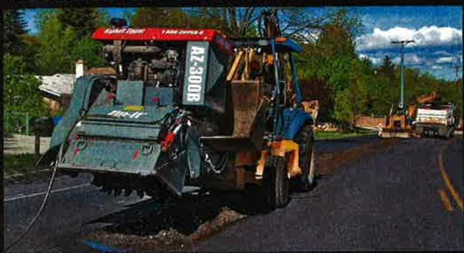
*"We're able to grind a 1000 feet long ditch 9 feet wide in 2 hours to get ready to excavate. It would normally take us 2 days!"*
