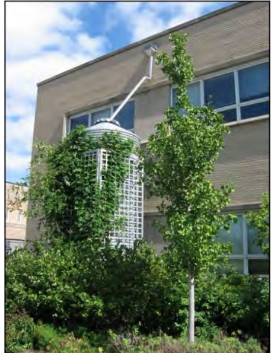
Distributed Site Design Measures, such as this cistern, can provide significant reductions in site runoff. Photo Credit – U.S. EPA
