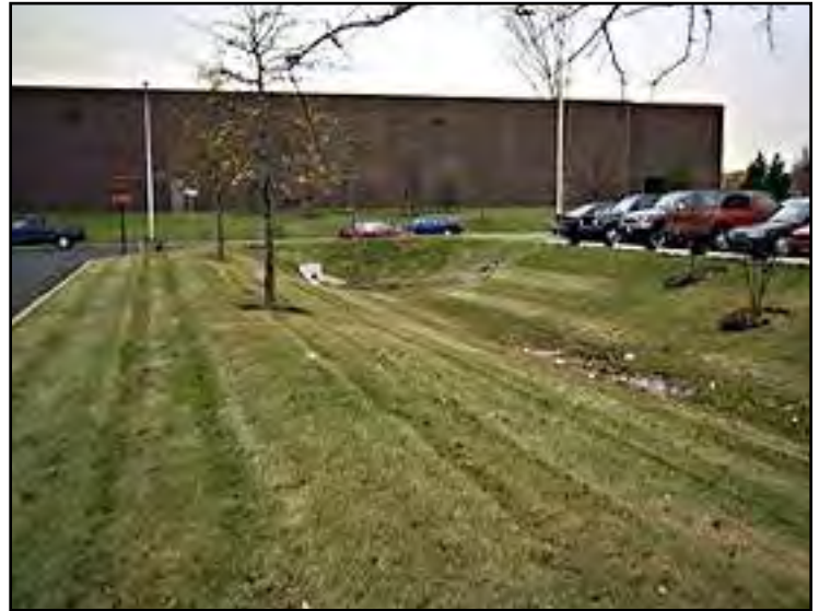
Grassed swale. Photo Source: EPA
