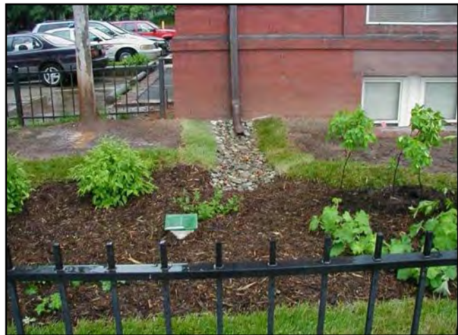
Roof disconnection. Source: LID Center
