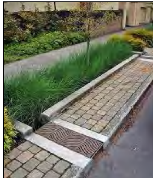
Roadside bioretention. Source: sitephocus.com
