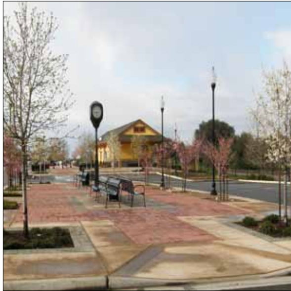
Refurbished Loomis Train Depot and Multi-Modal Transportation Center
