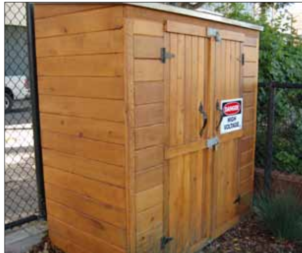
Enclosed Mechanical (2A.4)
