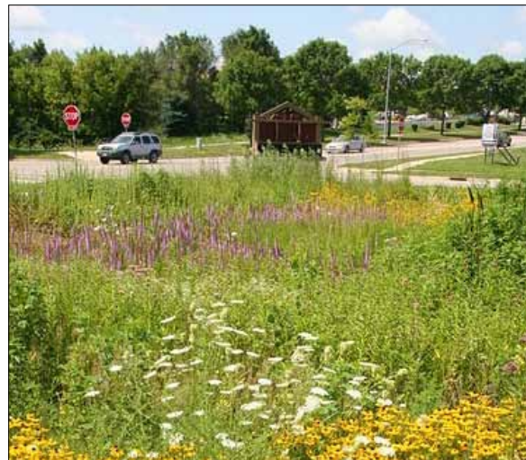
Rain Garden Stormwater Collector (2B.1)
