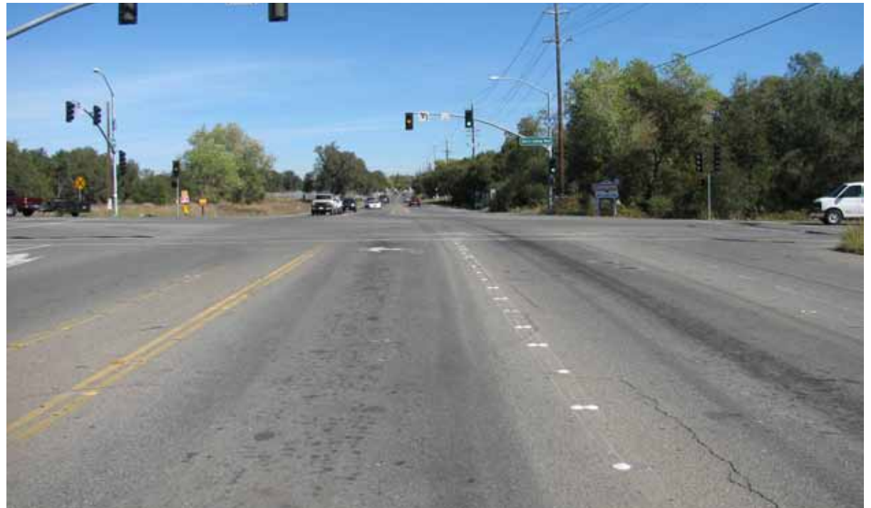
West Gateway Existing Conditions
