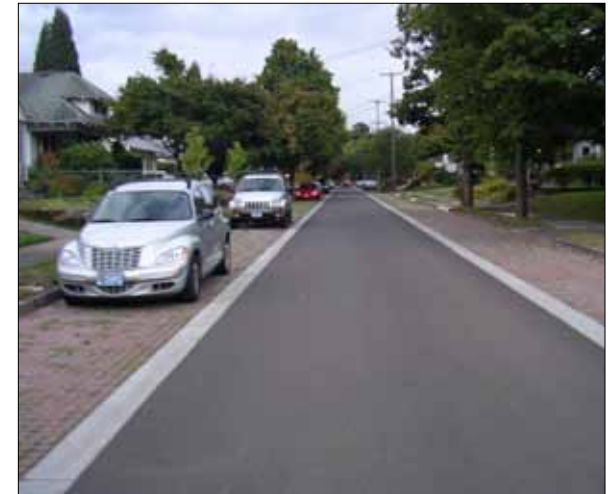
Permeable Pavers on Parking (1A.6)
