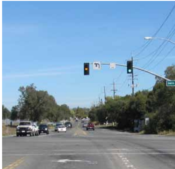
Unmarked Gateway at Sierra College Boulevard
