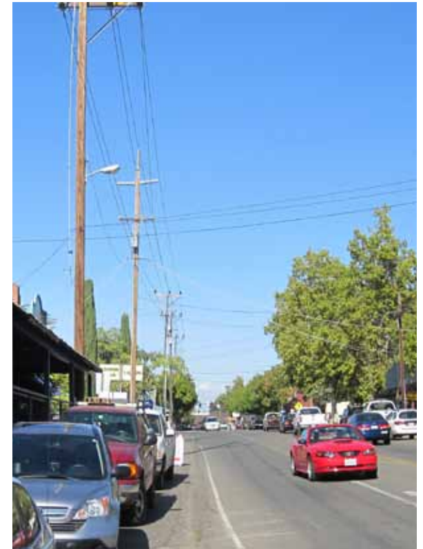
Overhead Electrical Wires to be Placed Underground
