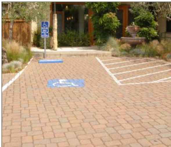
Traffic Calming Through Textured Paving (2C.2)
