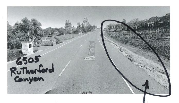
Dump grindings along edge of shoulder 100' or so apart. (To be spread by Town Crews) BOYINGTON ROAD (Paving Plan)
