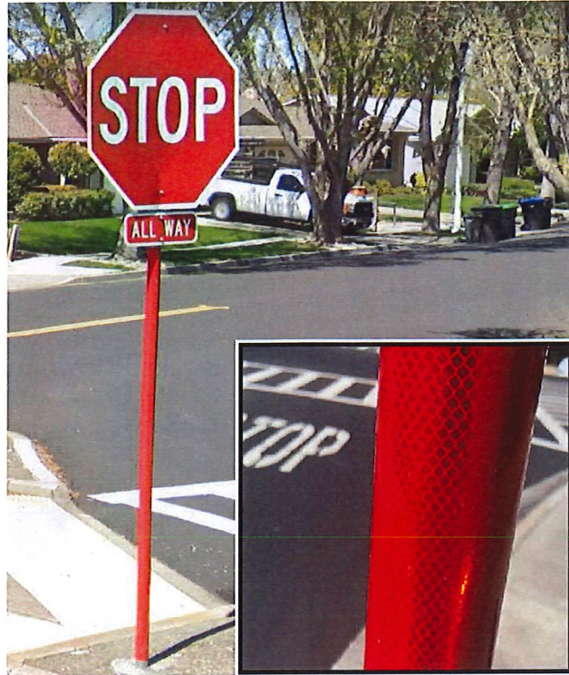
Permanent reflective red tape to be placed on stop sign pole
