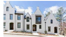
Serenbe, GA rowhouses - color and architecture too northern european for Loomis, but that could be tweaked
