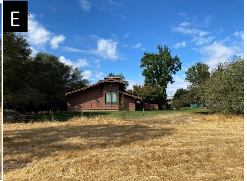
View E: Facing the rear of the Loomis Library & Community Learning Center that is neighboring the project site.
