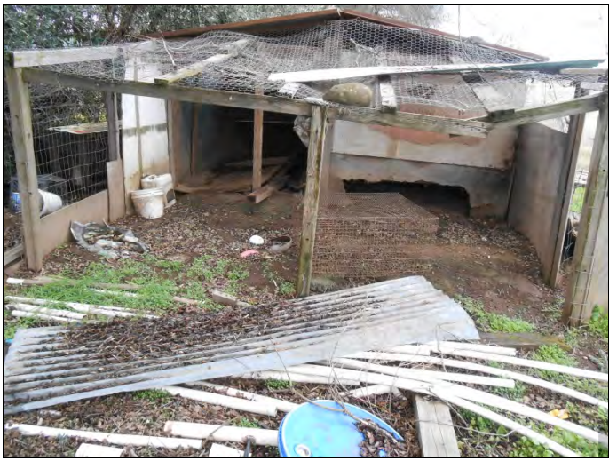
79. View of deteriorated shed at northeast area of subject property along facing west
