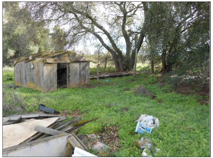
80. View of deteriorated shed at northeast area of subject property along facing southeast
