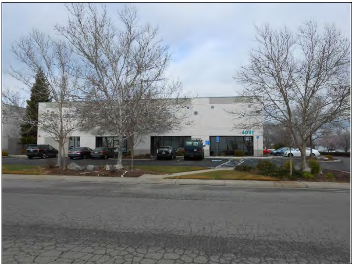
99. View of commercial building at 4041 Alvis Court south of subject property facing north-northwest
