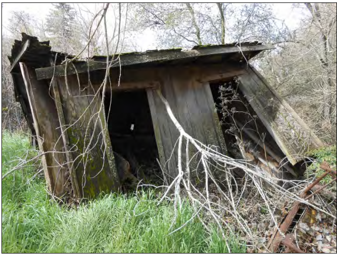
25. View of former well and shed/pumphouse near west boundary of subject property
