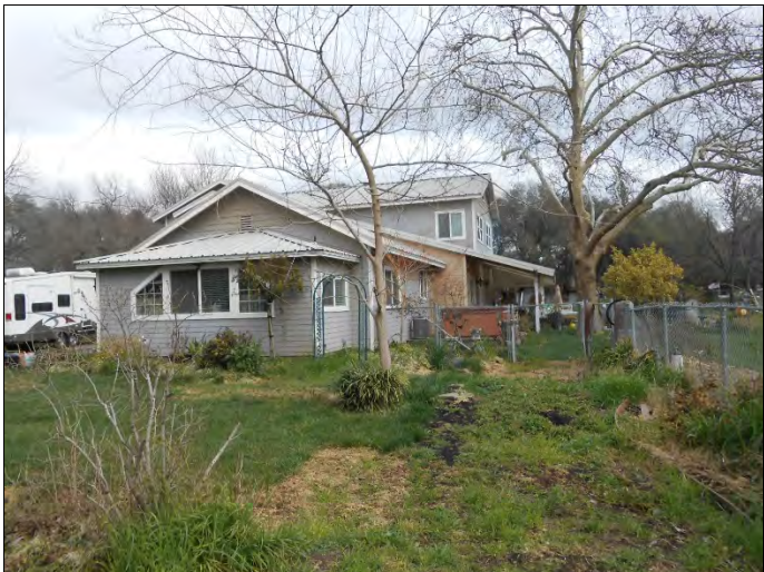
105. View of residence at 3969 Bankhead Road east of subject property facing east
