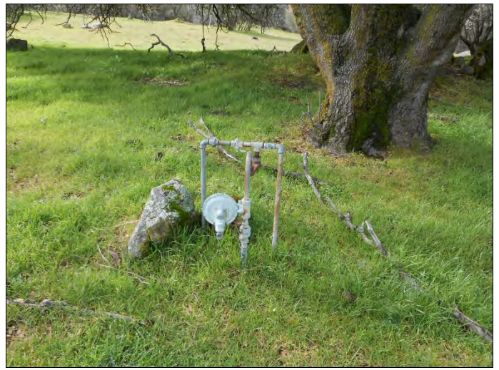
32. View of abandoned natural gas utility line in central area of subject property
