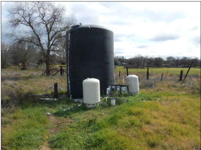
75. View of water storage tank at northeast area of subject property facing southeast
