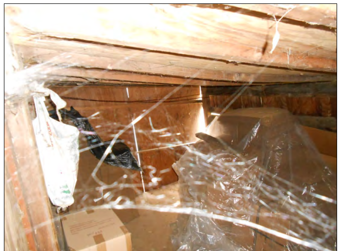
84. View of interior of storage shed
