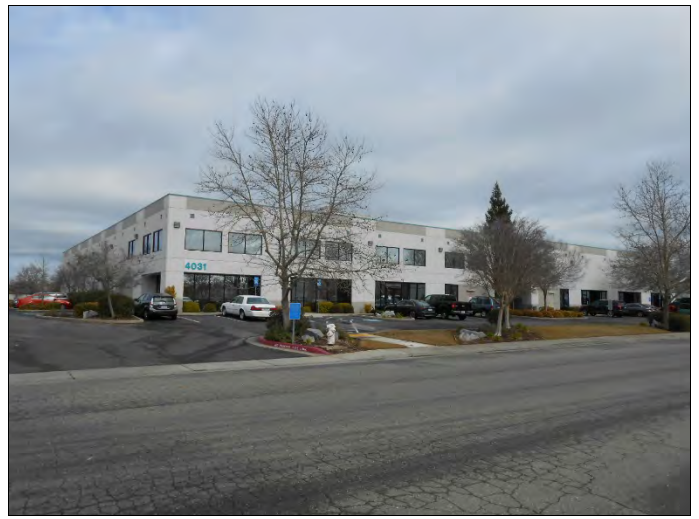
98. View of commercial building at 4031 Alvis Court south of subject property facing north-northeast
