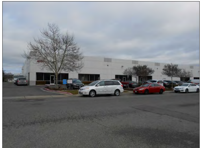
100. View of commercial building at 4051 Alvis Court south of subject property facing north-northeast
