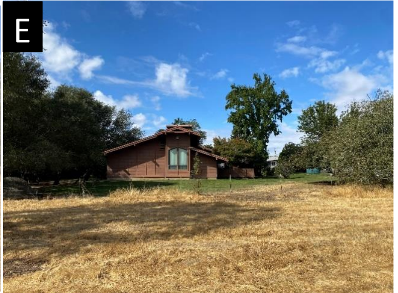
View E: Facing the rear of the Loomis Library & Community Learning Center that is neighboring the project site.
