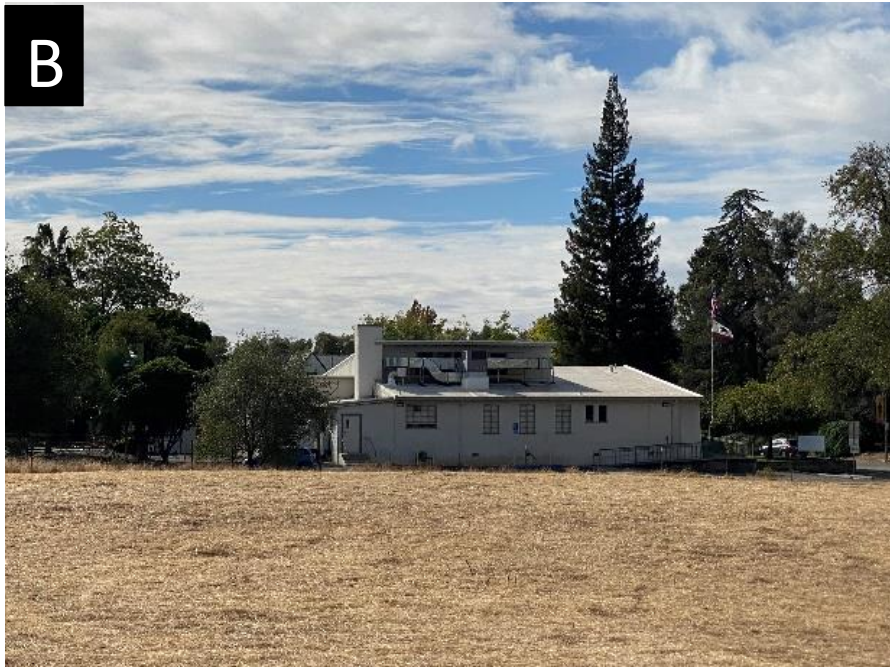
View B: Facing west along Horseshoe Bar Road towards Downtown Loomis.
