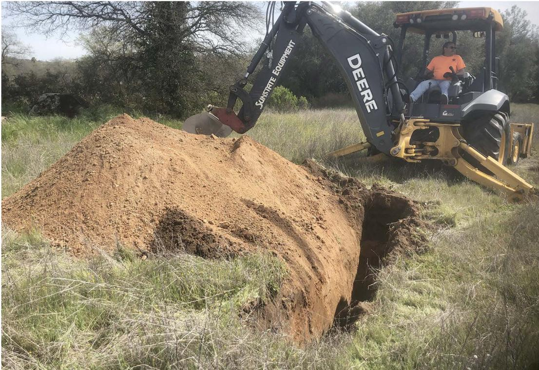
Photo No. 7 Typical Excavation Characteristics – Test Pit 17
