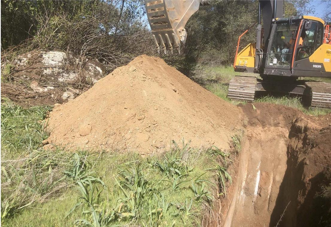
Photo No. 3 Typical Excavation Characteristics – Test Pit 4
