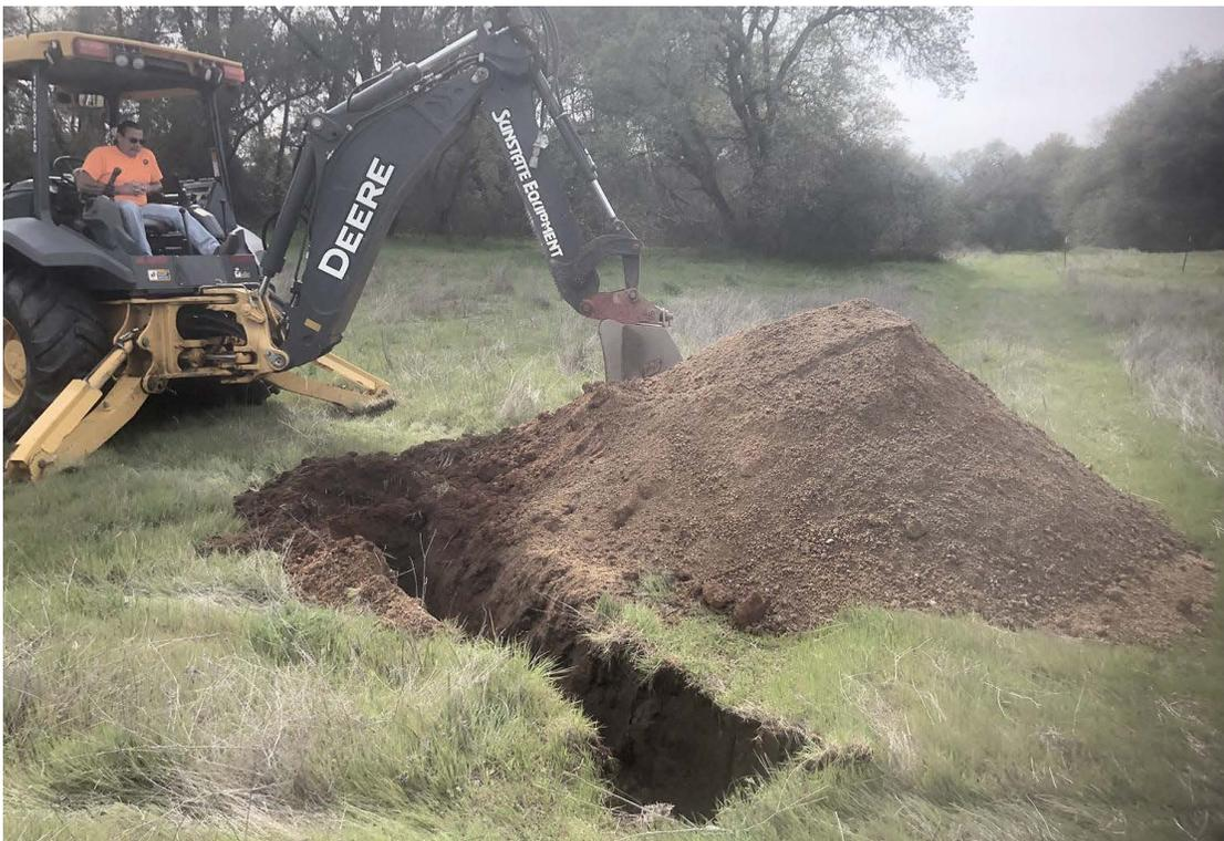
Photo No. 8 Typical Excavation Characteristics – Test Pit 20
