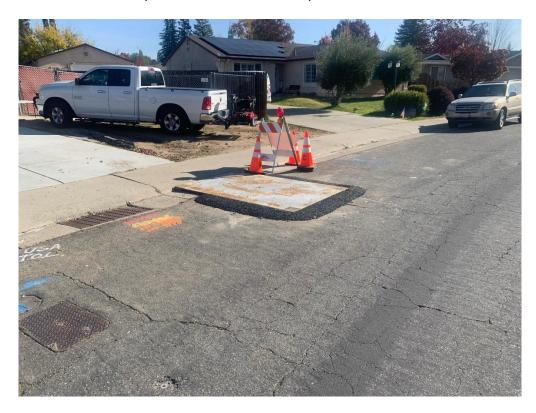
The scope of this project is to remove and replace approximately 24-feet of 18-inch RCP storm drain from the edge of the curb inlet to the edge of the manhole, as shown below. The line is dry, when there is no precipitation, so dewatering or bypass pumping is not anticipated. The invert elevation of the existing pipe is 2-1/2 feet at the curb inlet and 4-1/2 feet at the manhole.
