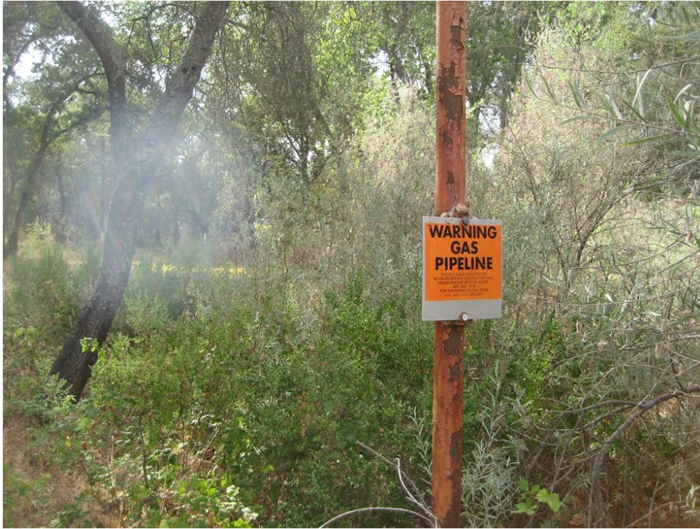
Photo 19: View of a natural gas pipeline marker located in the northeastern portion of the subject site.
