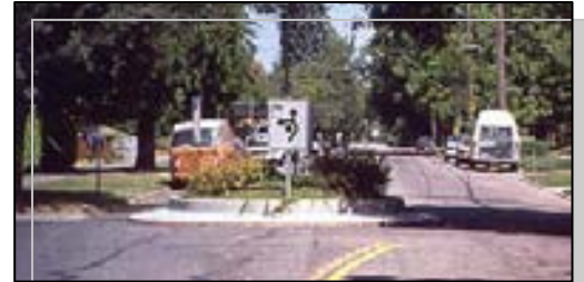
Example: Vertical inner curb and mountable apron.
