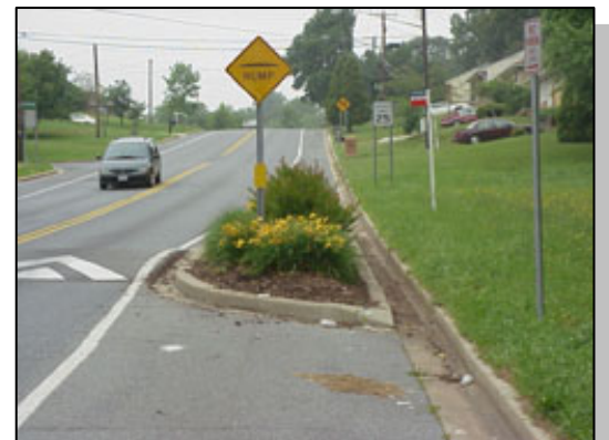
Example: Retrofit design with unimpeded drainage.
