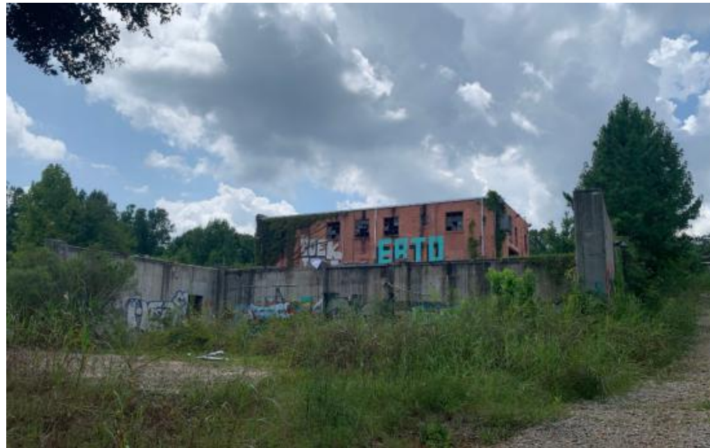
RETAINING WALL AND PLATFORM
