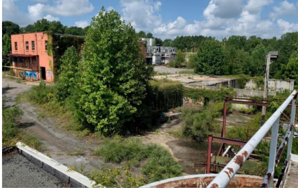
ELEVATED VIEW OF MILLING HOUSE
