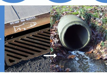
Storm drainage systems are designed to prevent flooding by collecting stormwater when it rains. This stormwater flows over surfaces, picks up pollutants, and eventually discharges into lakes, streams, and rivers. Unfortunately, there is no treatment process in the storm drain system to filter out pollutants before they reach downstream waters.
