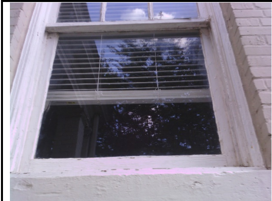
Exterior Side B Wood Trim
