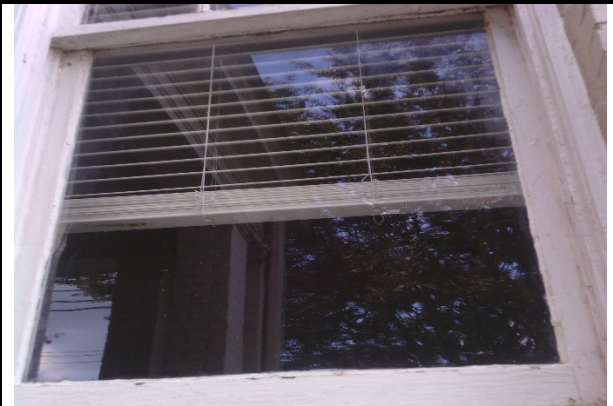
Exterior Side B Wood Trim
