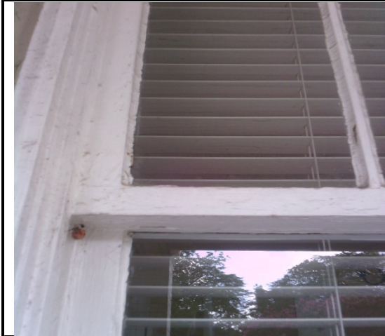
Exterior Side B Window Sash
