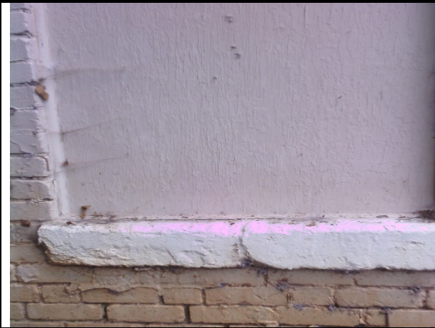
Exterior Side C Window Sill (concrete)
