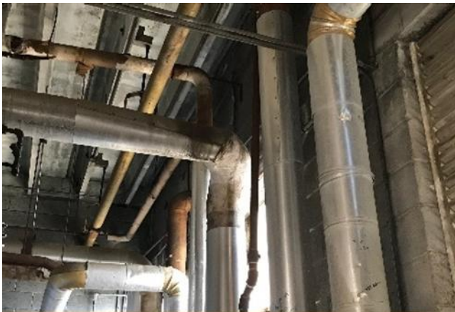
6" pipe elbow insulation
