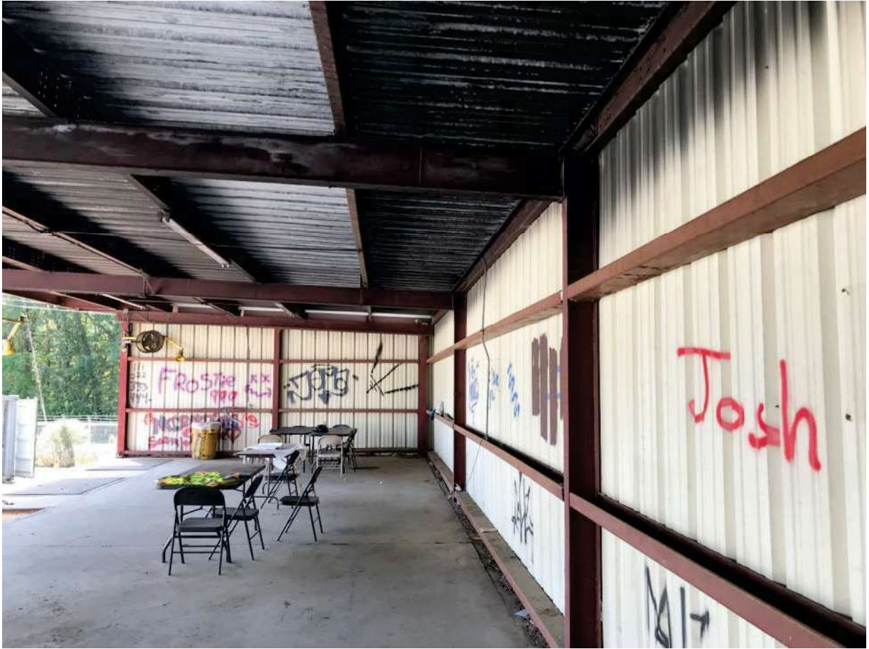
Image 4: Building 3 interior looking South.
