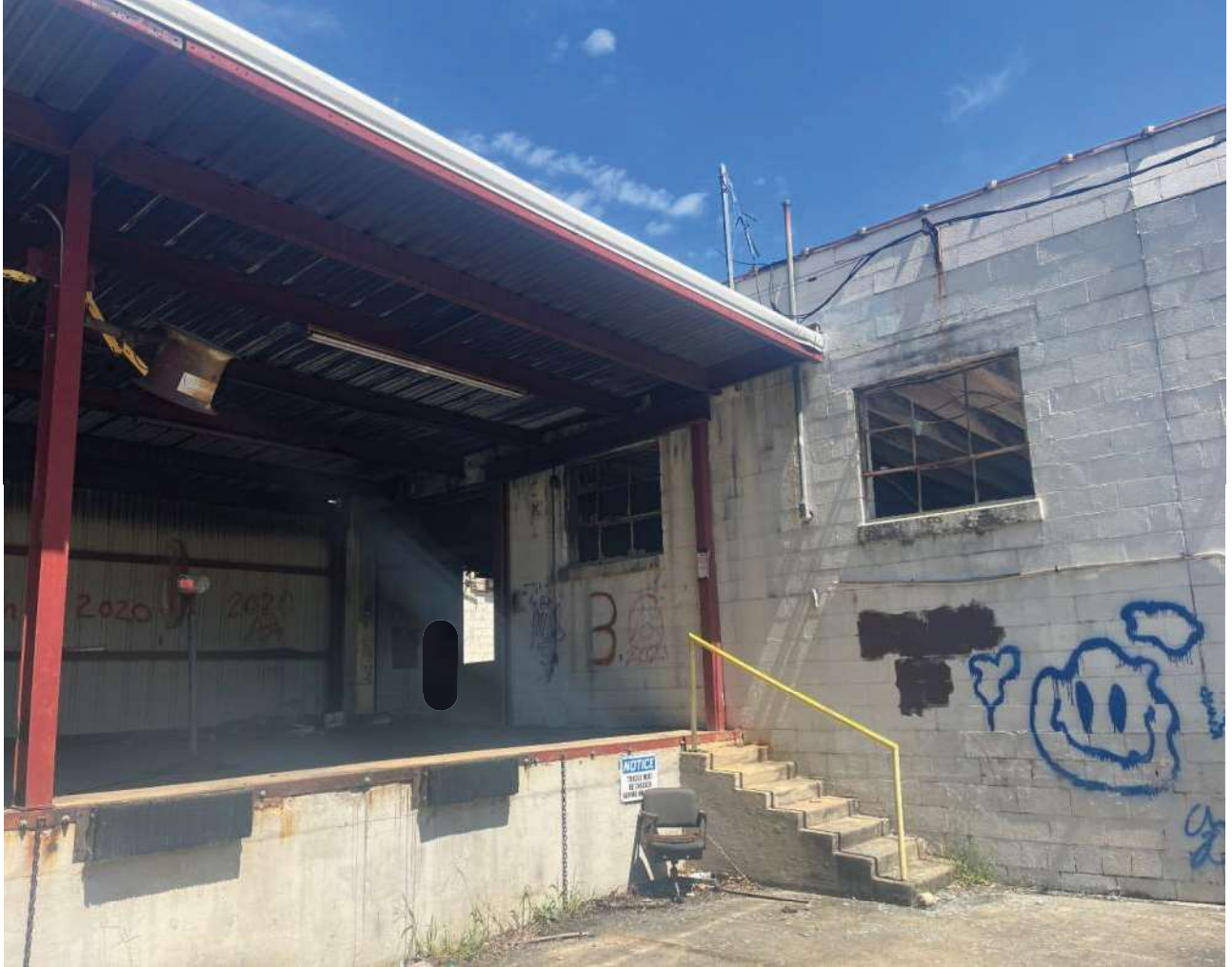
Image 1: Eastern elevation of loading dock structure at Building 3
