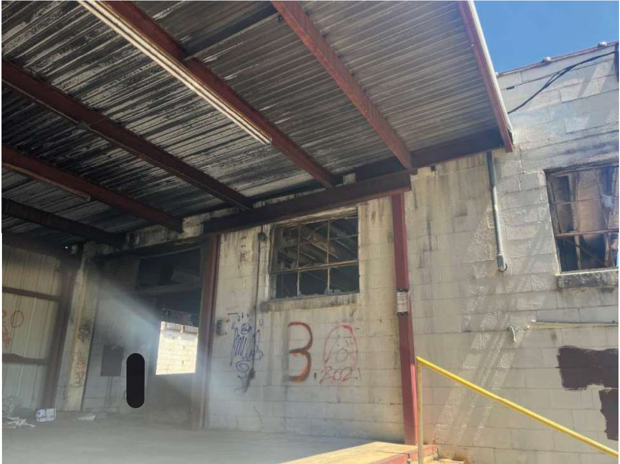
Image 2: Building 3 connection to existing block building.
