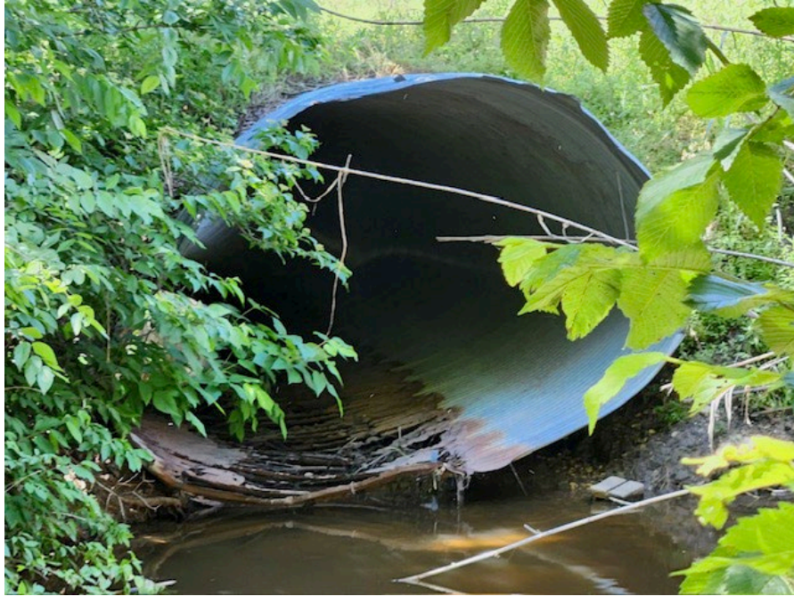
Pictures of Culverts at Lewis Lane
