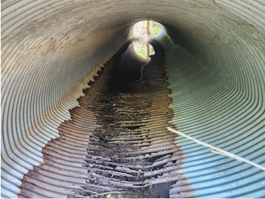
Pictures of Culverts at Lewis Lane
