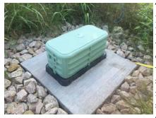
There are approximately 90 dead-end water lines throughout the City. These dead-end lines pose a water quality issue, because water can become trapped, and the residual chlorine levels can drop adversely impacting water quality. The City is actively flushing and/or testing these dead-end lines each month. Soon the city will start installing automatic flushing valves (AFV). These devices are in use on the end of the water
