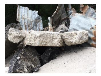
The east bridge has been demolished. As was suspected, there was no reinforcing steel in the deck. More concerning was the fact that the deck was not connected to the beams and girders. During the past flooding events, the deck had floated four inches to the south.
