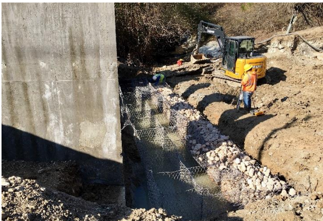
West Bridge Gabions
