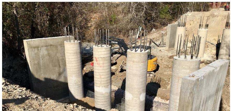
West Bridge Retaining Walls and Drill Shaft Columns
