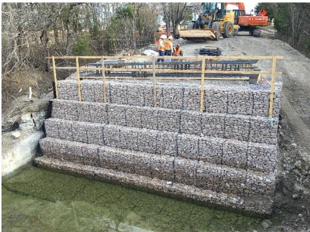
West Bridge North Side Gabions
