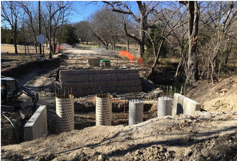
East Bridge Looking West
