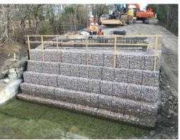
Things are moving along at the Blondy Jhune bridges project site. Most of the work has been completed on the abutments, retaining walls, and gabions on the south side of the west bridge. The abutment cap and retaining walls are not finished yet on the north side of the west bridge.
