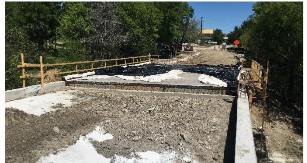
West Bridge Looking North
