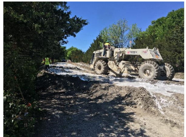
Blondy Jhune Road west of the West Bridge Looking West
