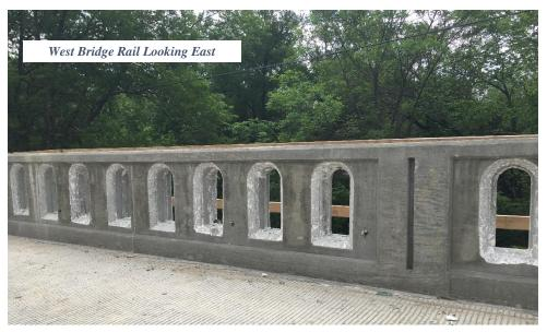
The rails are finished on the west bridge. The white residue visible in the arched openings is from the slip forms used to create the arches. This is kind of like buttering the pans so that the eggs don't stick.
