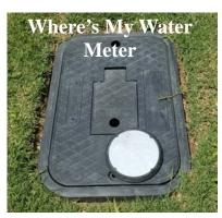
Your water meter is located outside typically in your front yard in a black box with a transmitter (the round white button on top). Should there ever be a leak that needs to be repaired, City staff will need access to your water meter and transmitter to allow the City to effectively make repairs. Its best that vehicles are not parked over or near your water meter box blocking access. Please do not cover the meter box with soil or do anything that would impede access.
