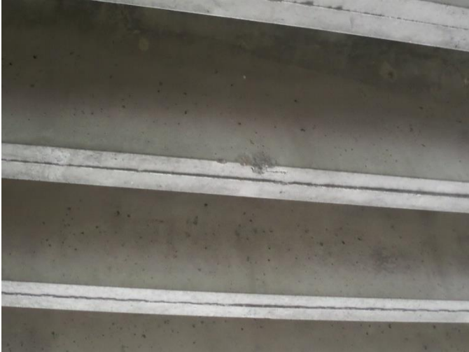
6" X 3" X 1" Spall at beam 10 7' from bent 2
