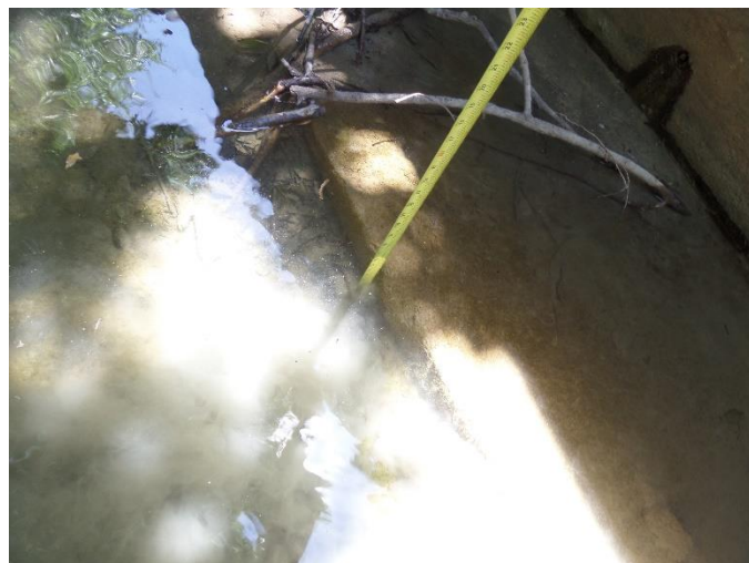
5" scour at bottom slab toe, northeast corner
