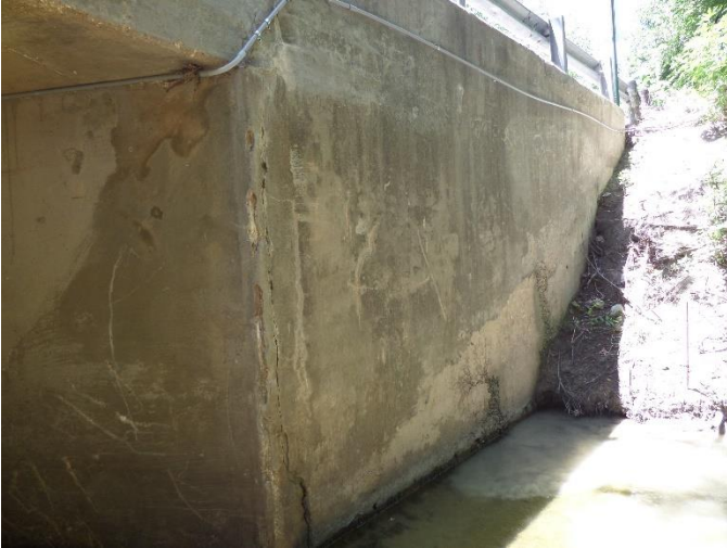
28: Abutment 1 – Northwest corner
