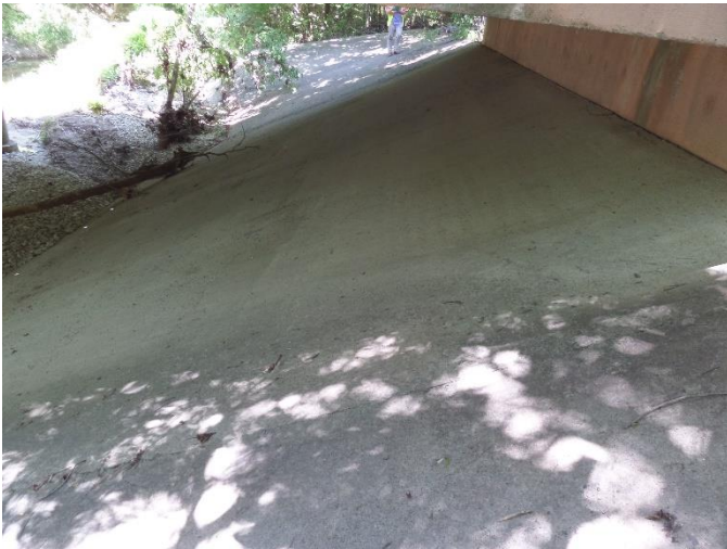
Typical – no deficiencies noted
