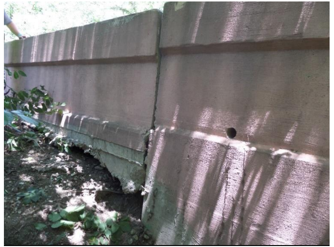
Scour and undermining both sides
