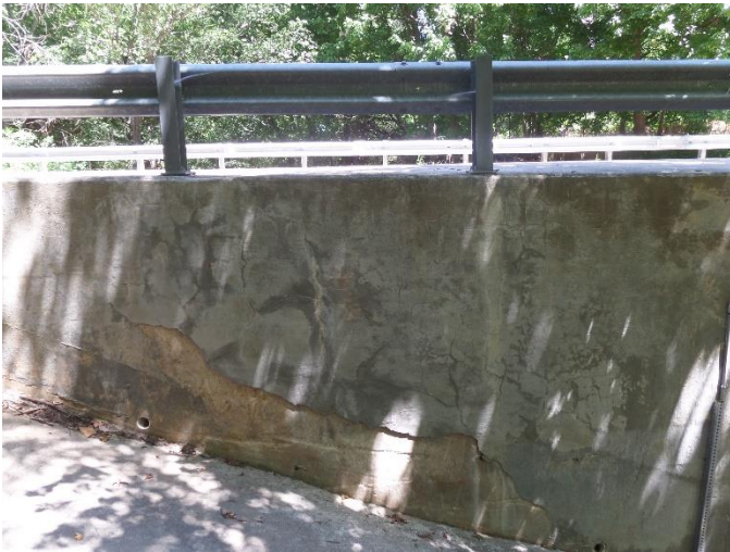
75% delaminated on southwest face abutment 1
