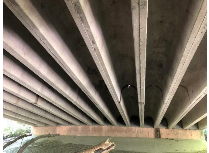
Longitudinal cracking under deck span 3 (Typ.)
