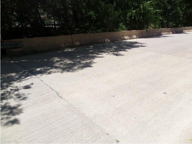
Southwest corner approach slab settled 1"
