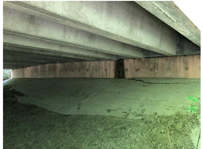
25: Abutment 2 – Looking Northwest
