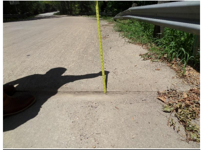
Approach slab settled 1" at roadway
