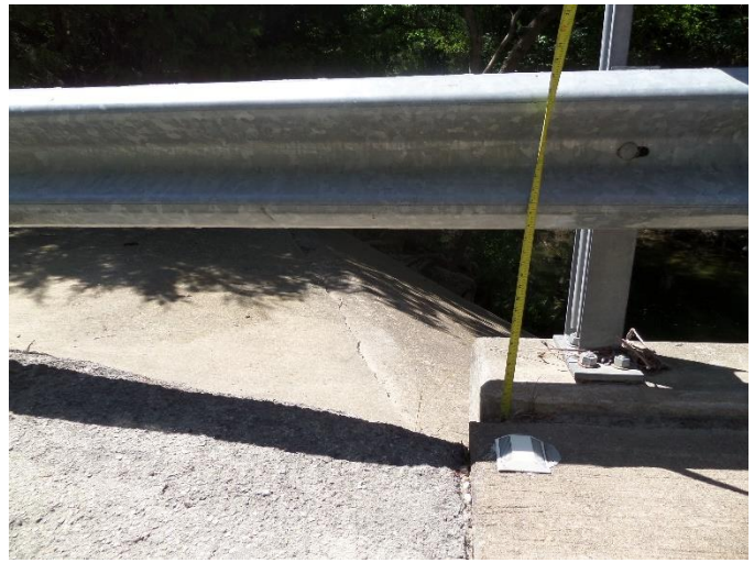
2-1/2" settlement of approach slab 2
