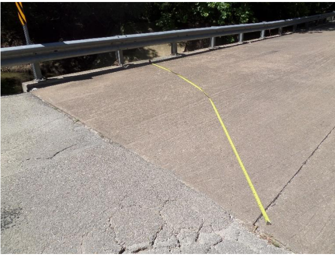
1/8" diagonal crack
