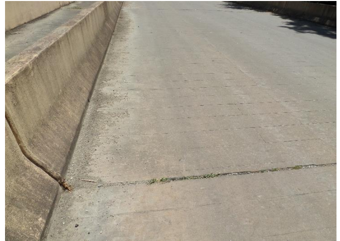
Shrinkage cracking along deck (Typ.)
