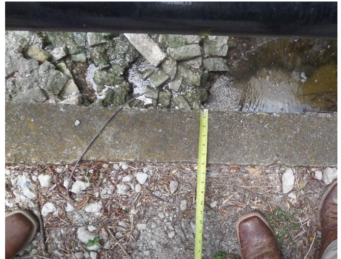
Headwall thickness varies from 6" to 8"
