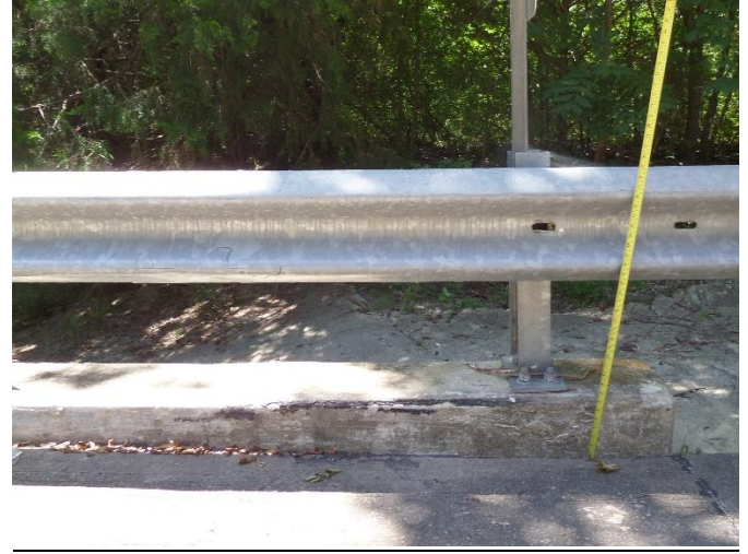
6" settlement of approach slab in southwest corner
