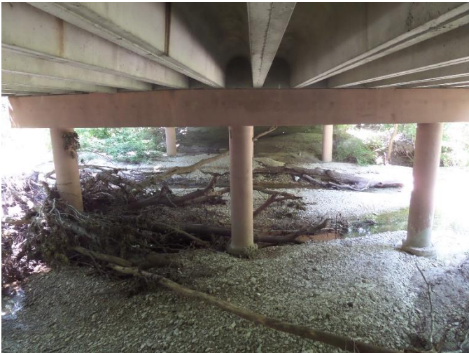
Evidence of flooding
