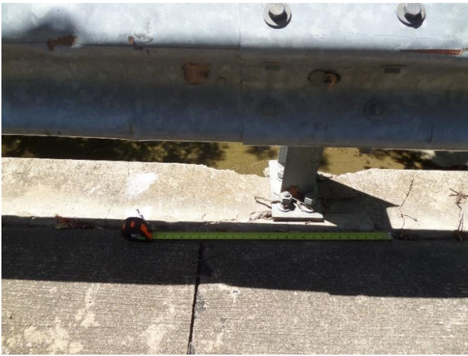
7" x 24" x 3" spall at the second post of span 2
