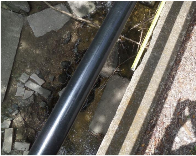
10" x 4" x 1" Spall midspan
