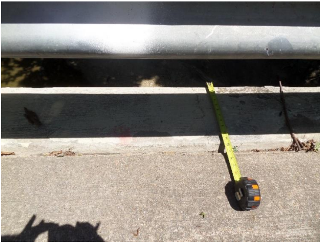
Full width hairline crack at the beginning of span 3
