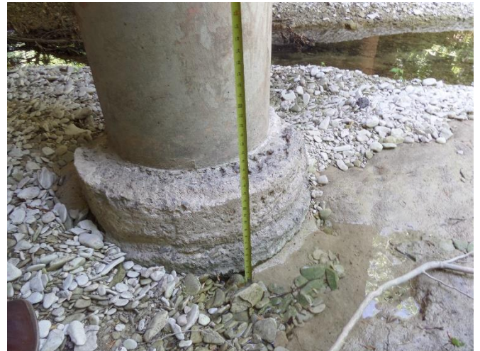
Exposed drill shaft from scour 13" (Typ.)
