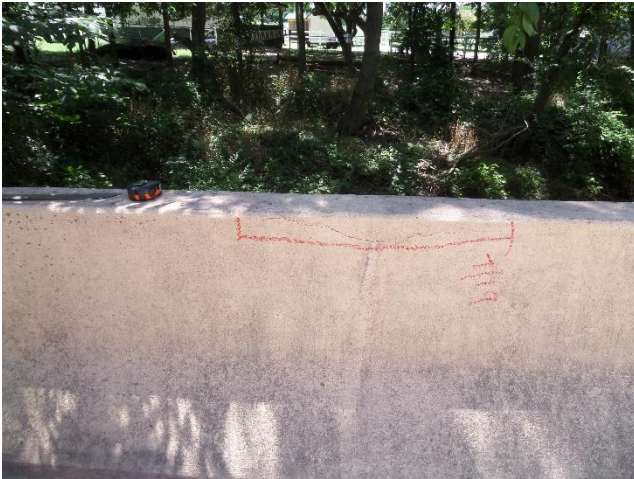
0.035" + 27" crack left railing span 1 at 12'
