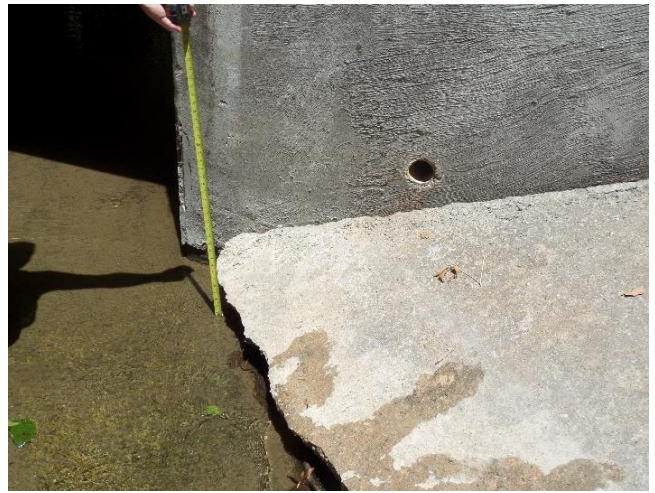
Toe exposed; chipping and undermining of riprap
