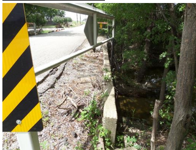
Headwall 2 out of plumb
