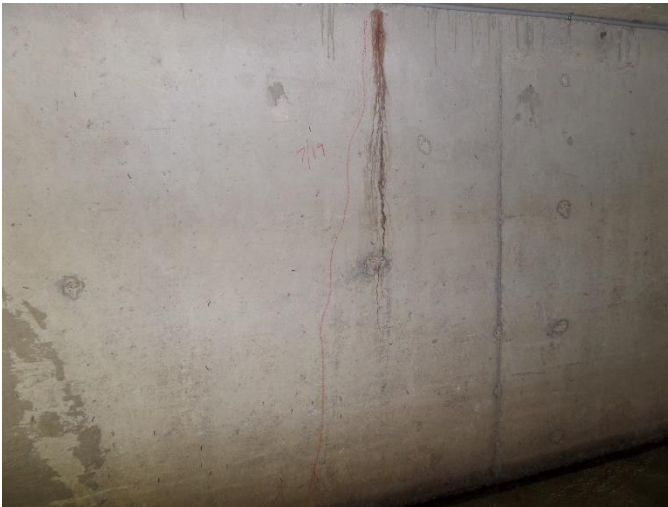
0.010" crack full height at 10' with efflorescence
