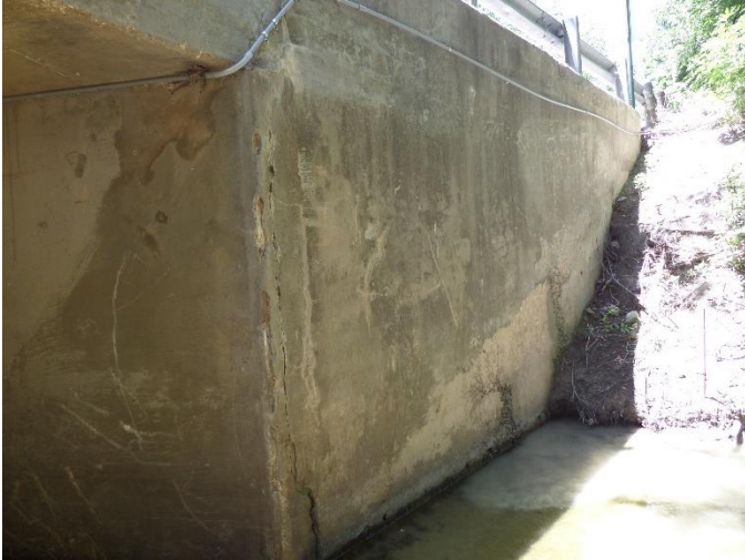
28: Abutment 1 – Northwest corner
