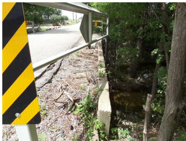
Headwall 2 out of plumb
