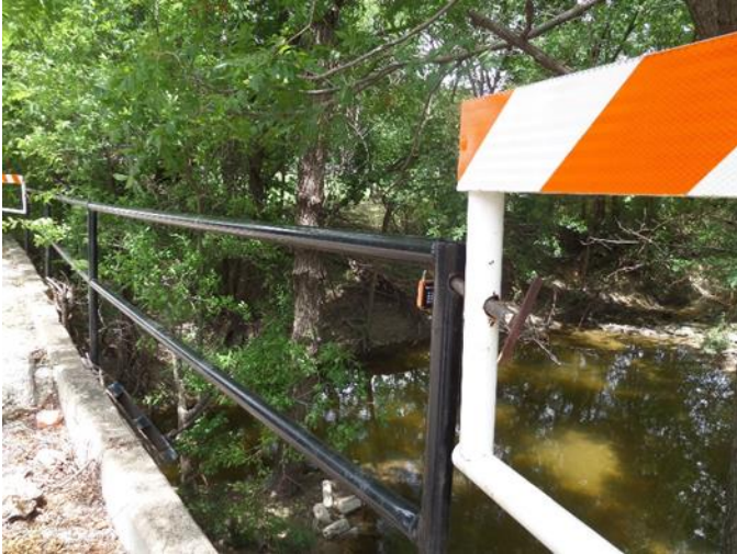
Railing/gate connection in good condition
