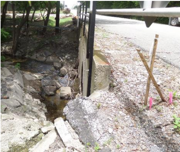
Typical - no deficiencies noted.
