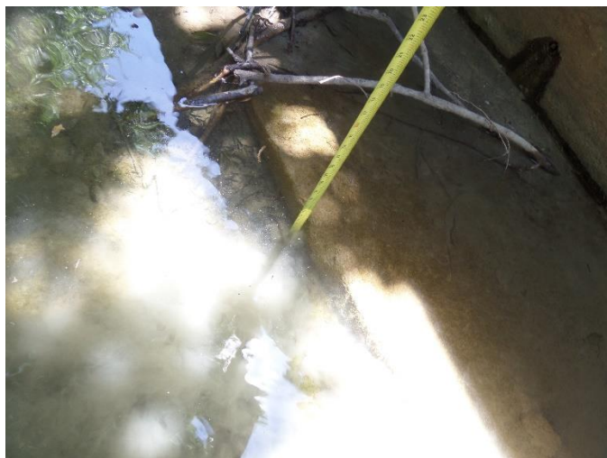
5" scour at bottom slab toe, northeast corner
