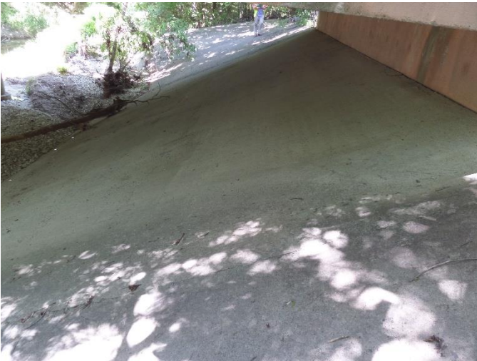
Typical – no deficiencies noted
