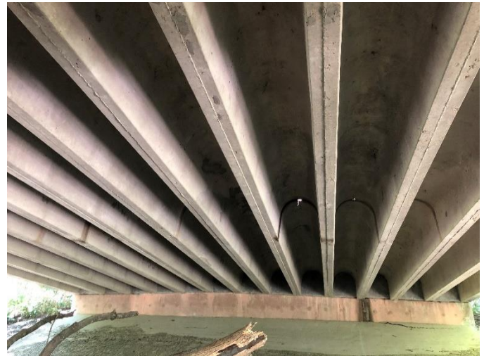
Longitudinal cracking under deck span 3 (Typ.)
