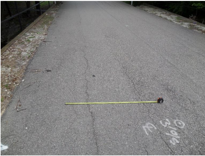
Left lane with Marginal longitudinal cracking (Typ.).
