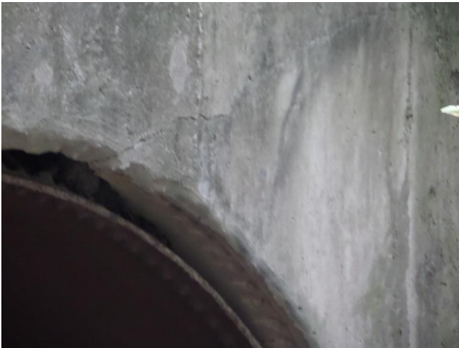
5' Horizontal crack near culvert 1
