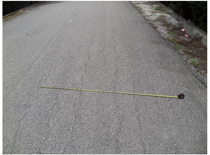
Right Lane substantial longitudinal cracking.
