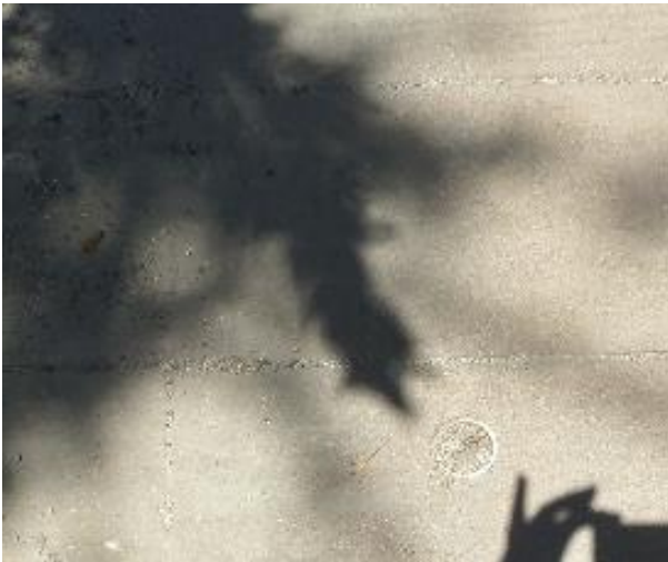
Scupper clogged mid span of span 1
