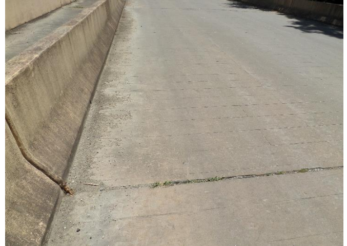
Shrinkage cracking along deck (Typ.)
