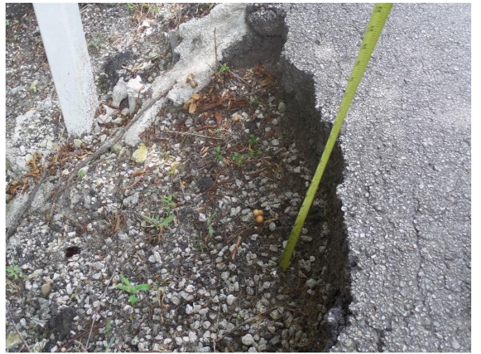
Substantial pavement failure (12")
