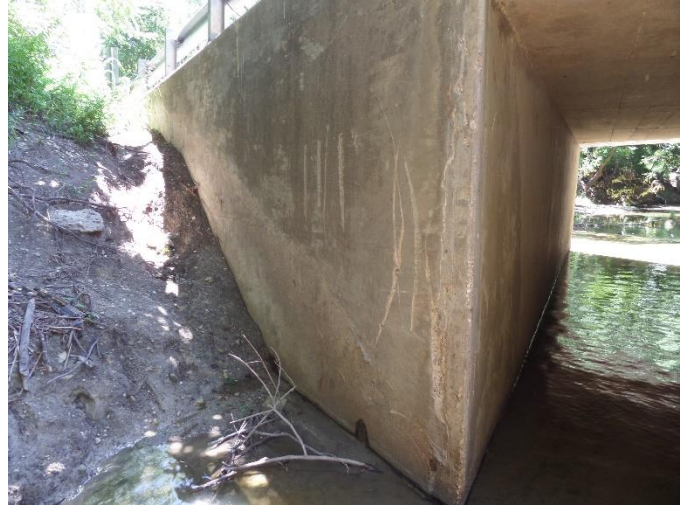
29: Abutment 4 – Northeast corner
