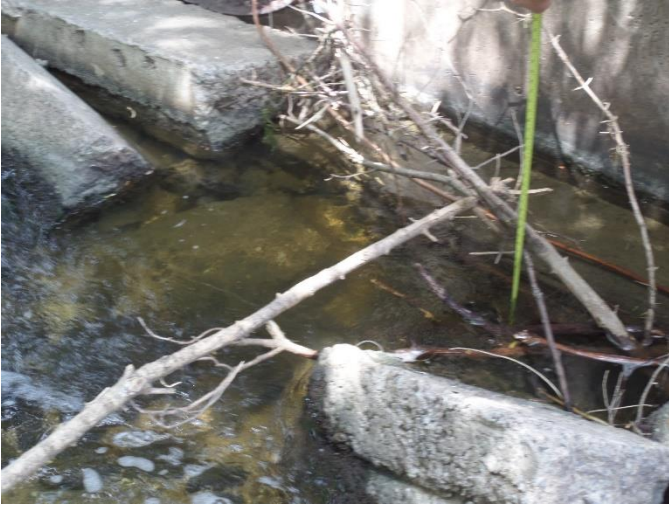
Undermining of headwall 1 at midspan
