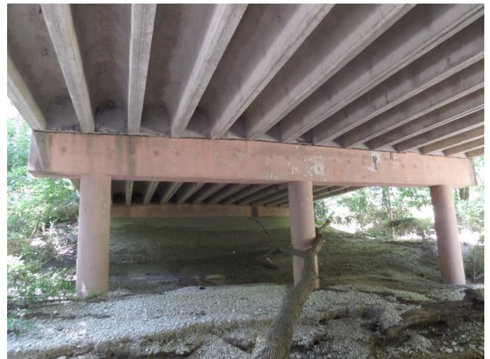
19: Span 2 – Under View – Looking North
