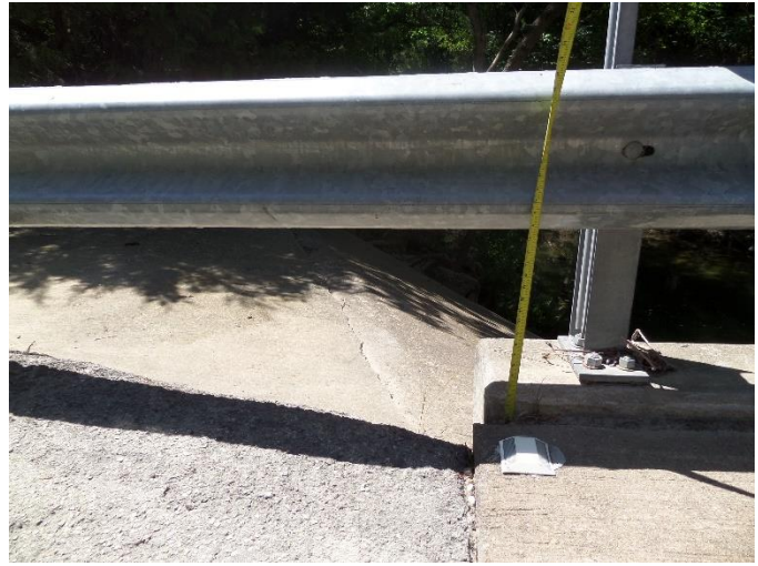
2-1/2" settlement of approach slab 2
