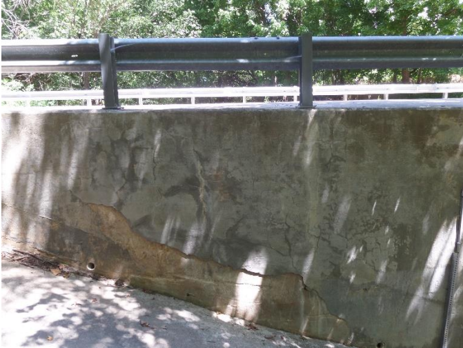
75% delaminated on southwest face abutment 1
