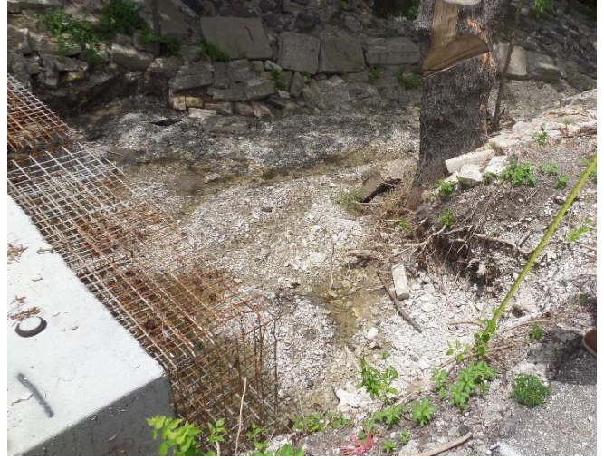
6' drop off 1' off the road (currently under construction)
