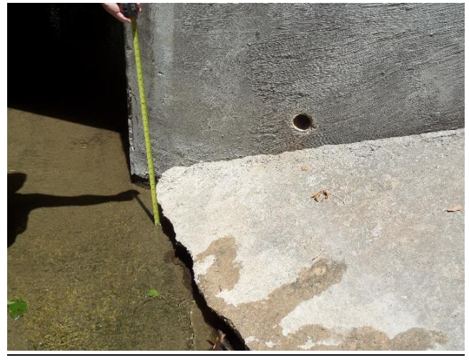
Toe exposed; chipping and undermining of riprap
