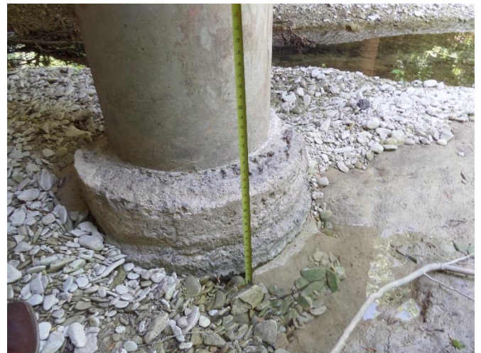
Exposed drill shaft from scour 13" (Typ.)
