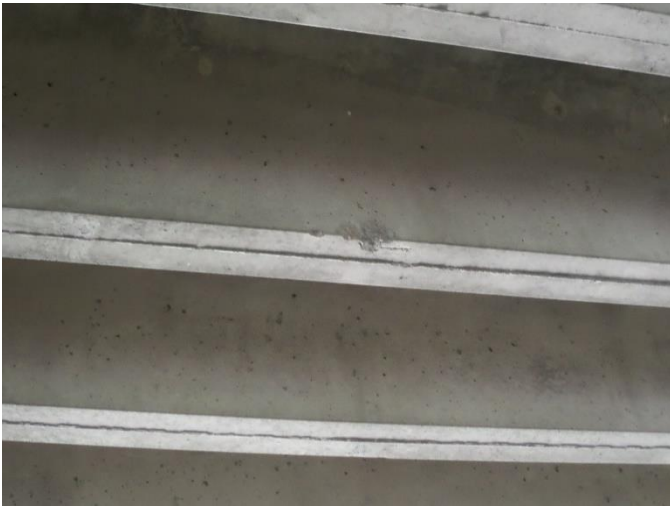
6" X 3" X 1" Spall at beam 10 7' from bent 2
