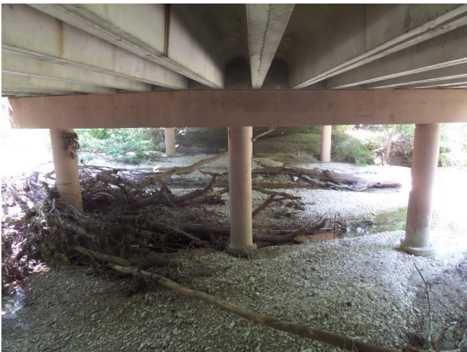
Evidence of flooding
