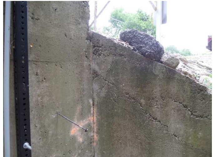
19" x 1/8" crack at wingwall 1
