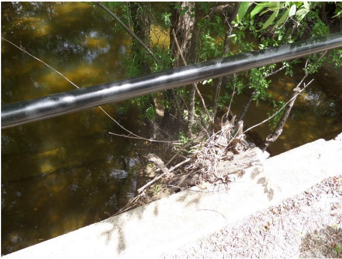
Evidence of flooding
