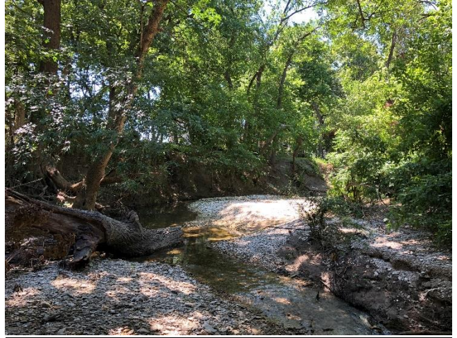
Typical – Slight bank erosion
