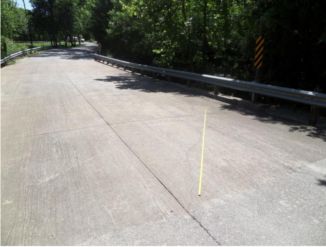
Diagonal crack at southwest portion of approach
