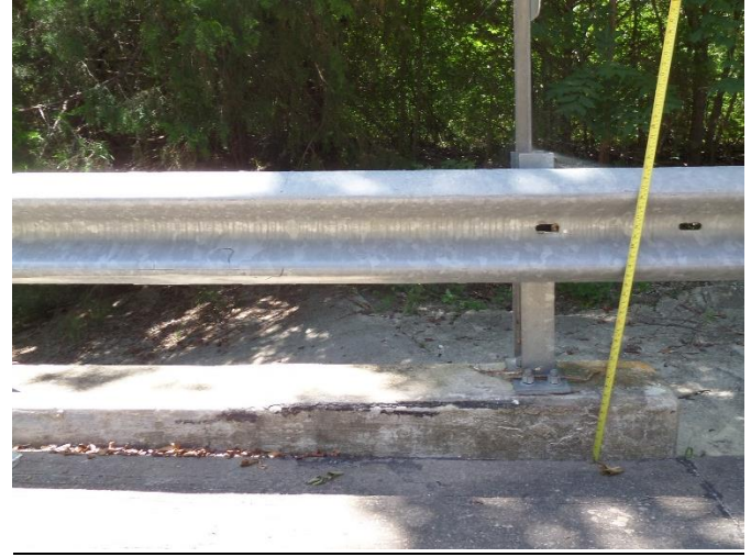
6" settlement of approach slab in southwest corner
