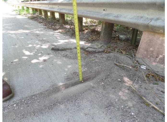
Southeast approach slab settled 1/2"
