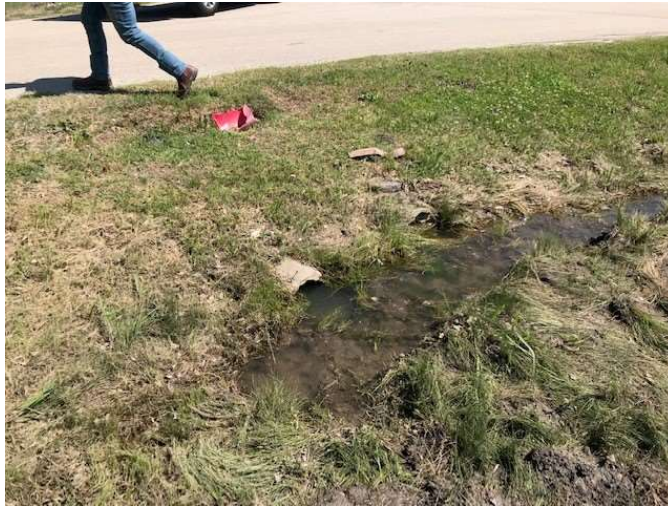
Image 1: Downstream Face of Mandarin Cove Culvert
