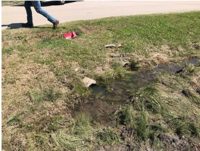
Image 1: Downstream Face of Mandarin Cove Culvert
