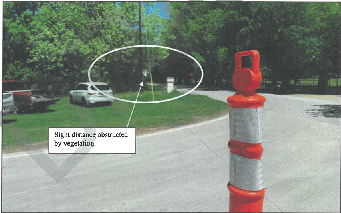
Figure 4: Sight Distance to the Left for Eastbound Blondy Jhune Road – Preliminary Field Visit
