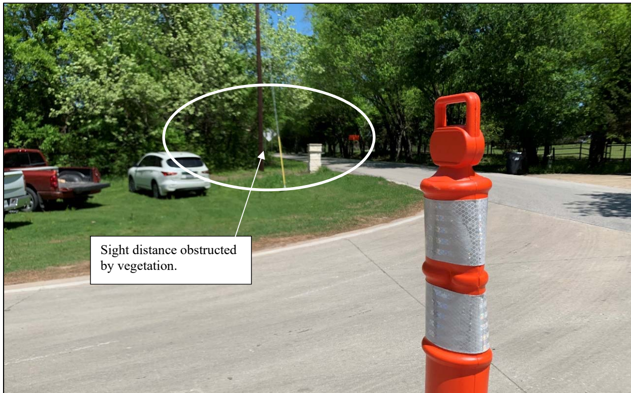
Figure 4: Sight Distance to the Left for Eastbound Blondy Jhune Road – Preliminary Field Visit
